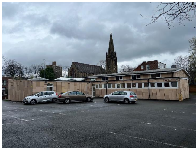
Rear elevation view from the car park
