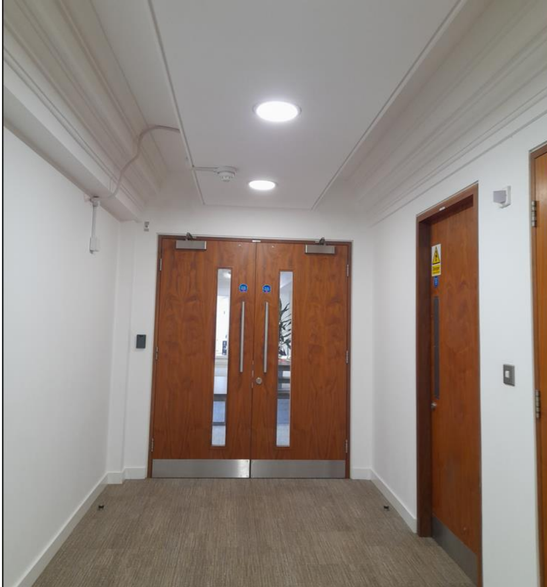
Figure 1. Showing corridor with cornicing and modern skirtings and doors.
