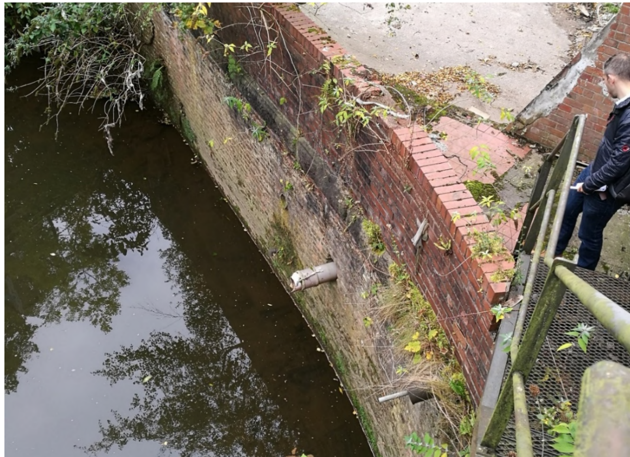
Figure 5-1 Existing Outfall Observed During Site Visit
