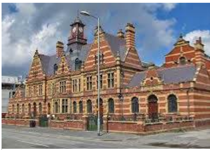
The front (Hathersage Road) block from the south-east.
