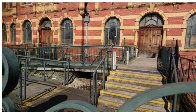
The ramp to the Females Pool entrance
