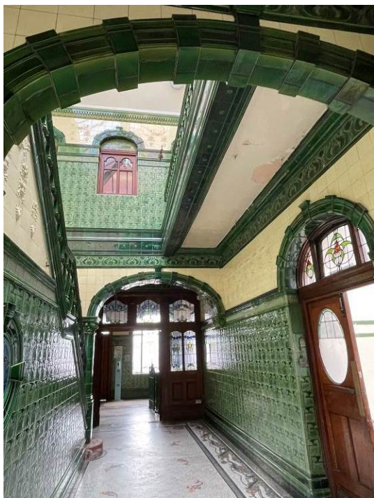
A wireless solution is proposed for historically sensitive areas with surviving finishes.
