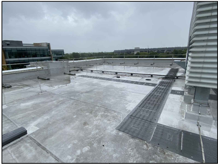
Area D Approximate area 55m 2 No. of PV panels 12 Output = 7.82kW p
