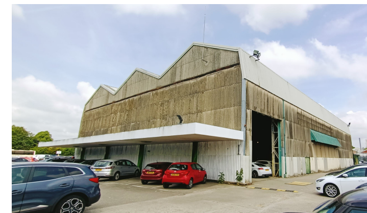
Warehouse View from South
