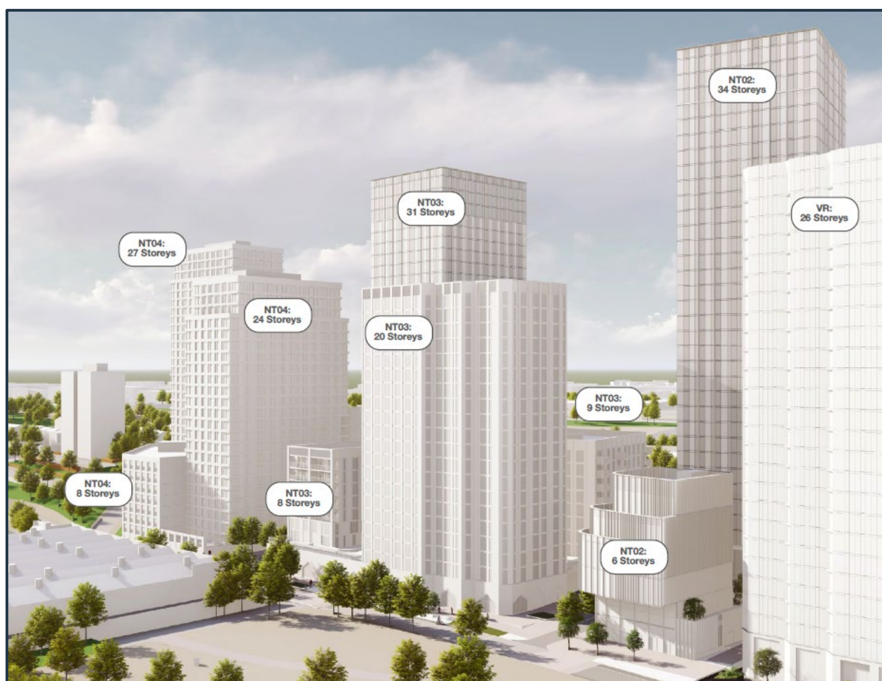
Figure 5.3: Building Heights Across Application 5 (NT02-04)
