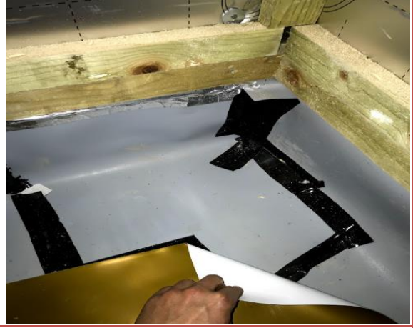
Verification of Service Penetrations-Good Condition
