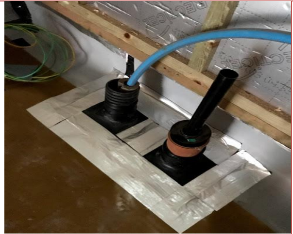
Verification of Service Penetrations-Good Condition
