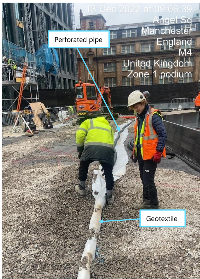
Figure 2-4 Perforated pipe installation in permeable paving system
