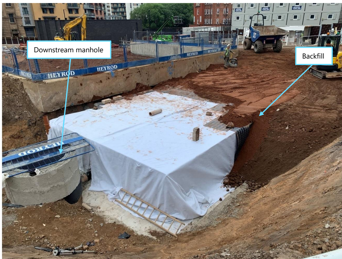
Figure 2-3 Backfilling on Attenuation Tank 1
