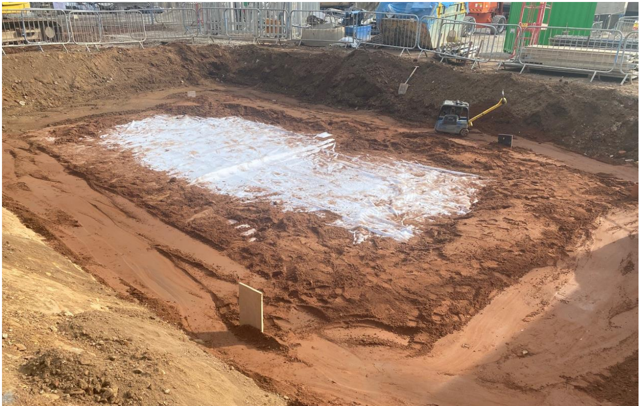
Figure 2-8 Backfilling of Attenuation Tank 2
