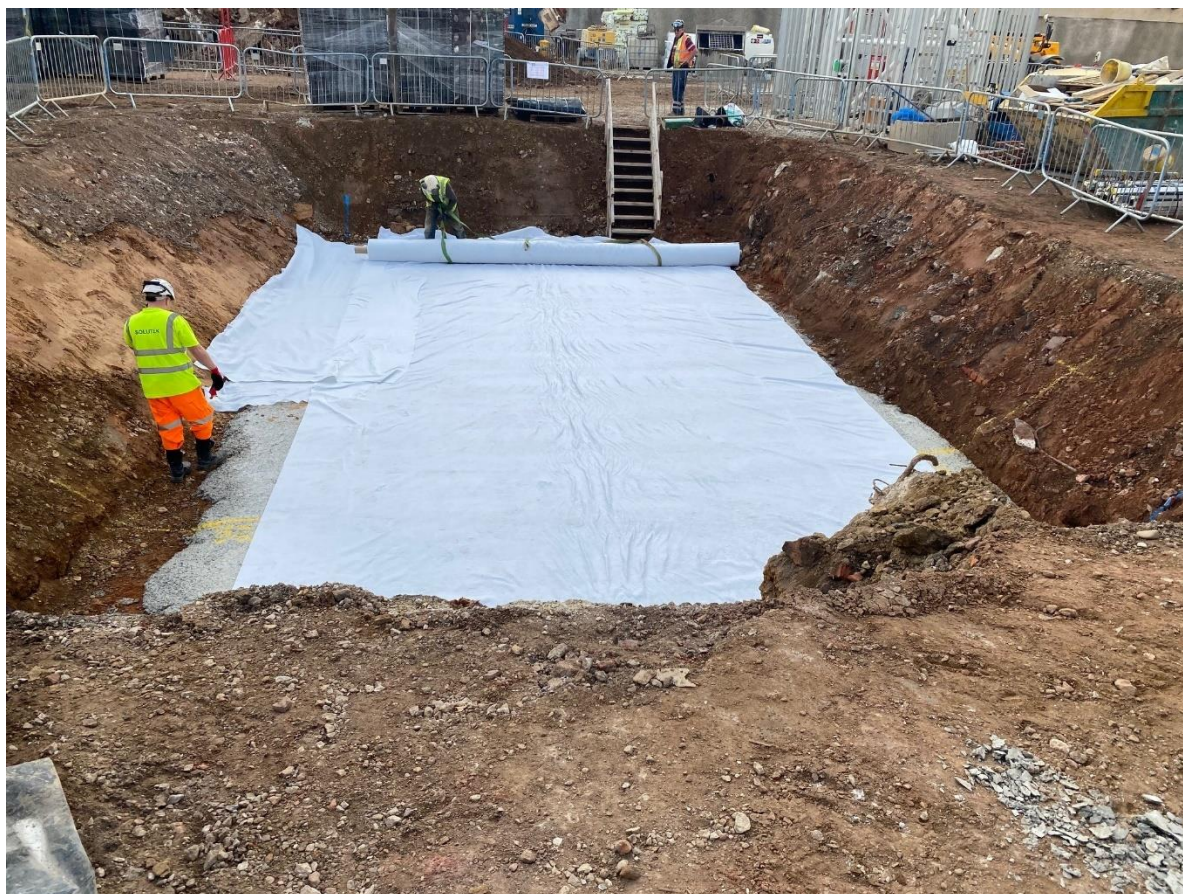
Figure 2-6 Ground preparation for Attenuation Tank 2
