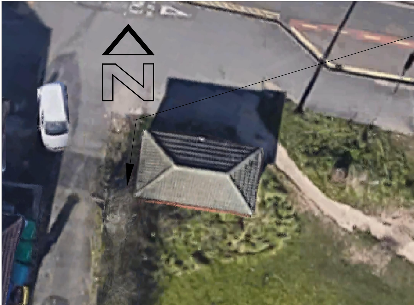
Existing Building in Location
