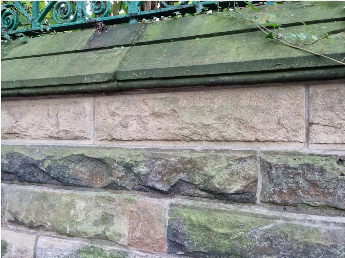
Photo 7: Historic wall repairs/replacement, new stones installed to top course of wall on Stenner Lane.
