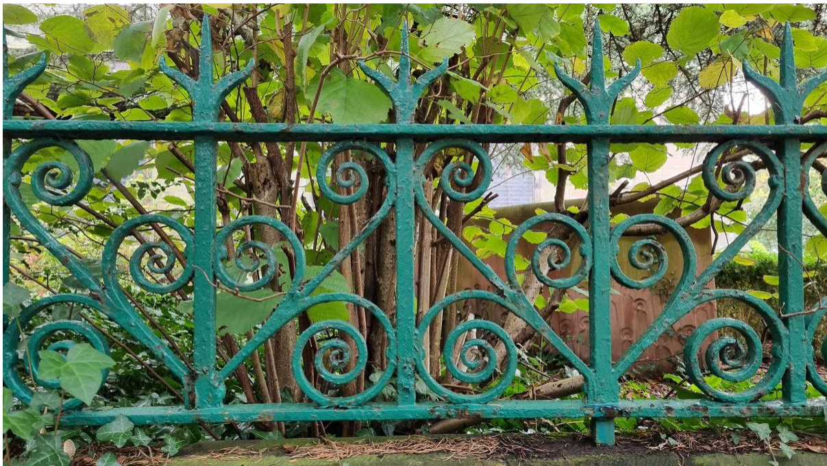
Photo 10: Existing cast iron railings fixed to coping stones on boundary wall at St James's Church/Stenner Lane.
