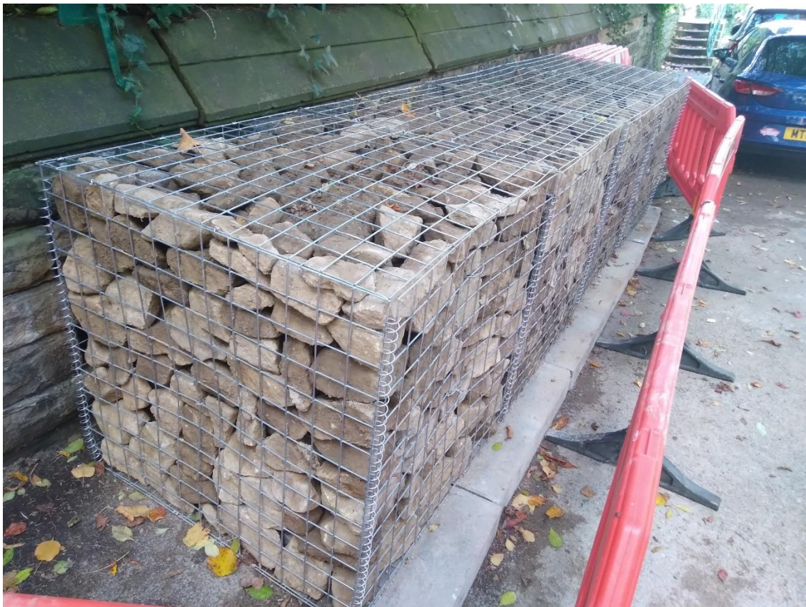
Photo 8: 4 [Nr] Gabion baskets installed adjacent boundary wall in October 2022.
