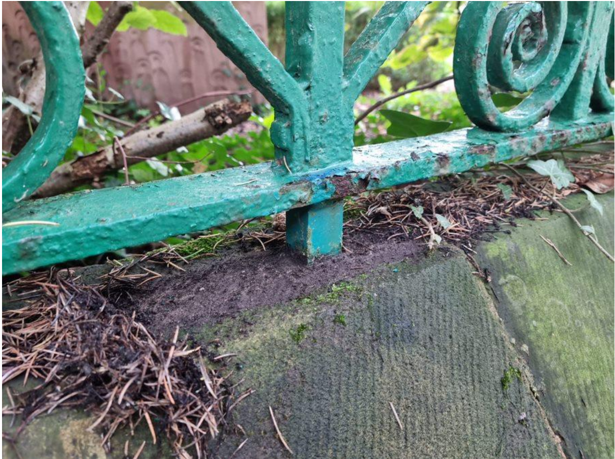
Photo 11: Existing cast iron railings fixed to coping stones on boundary wall at St James's Church/Stenner Lane.
