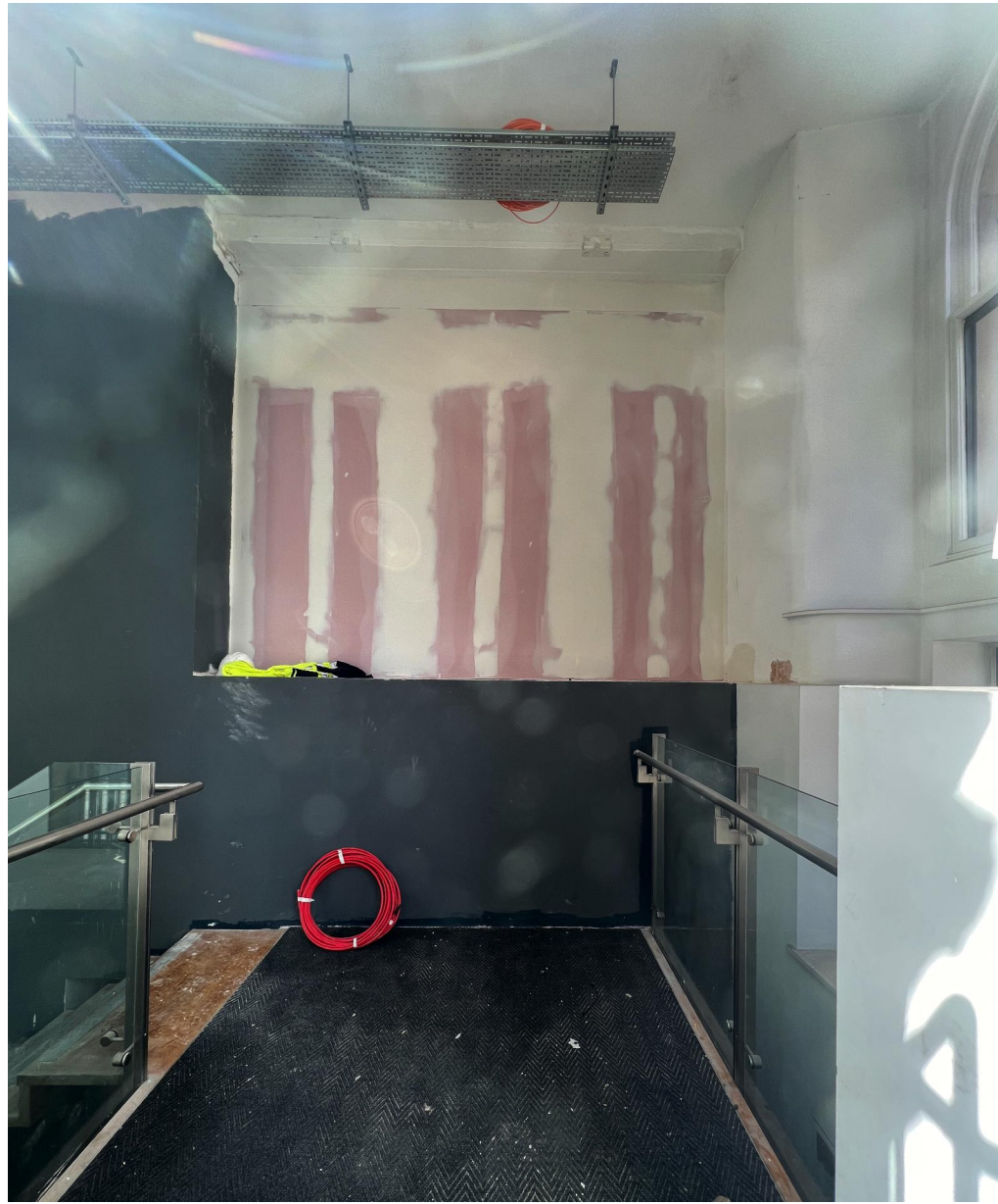
EXISTING ENTRANCE AREA
