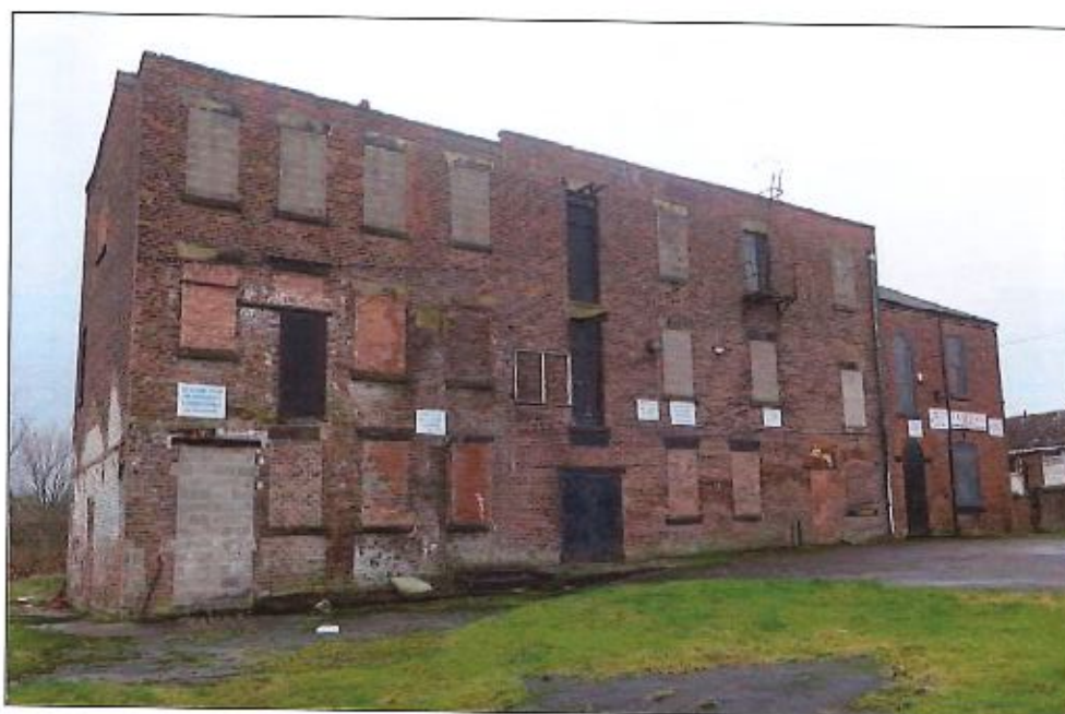
Figure 4. Central warehouse block demolished in 2019 as seen in 2017.
