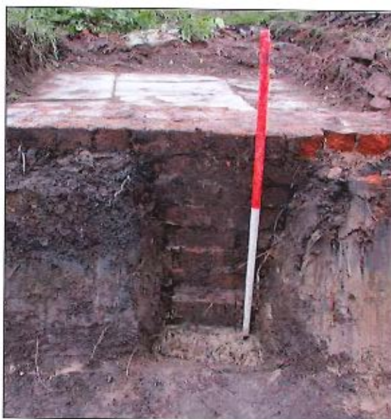
Figure 28. Sondage cut against western face of wall 006 showing foundation course and depth of natural clay. Looking east.
