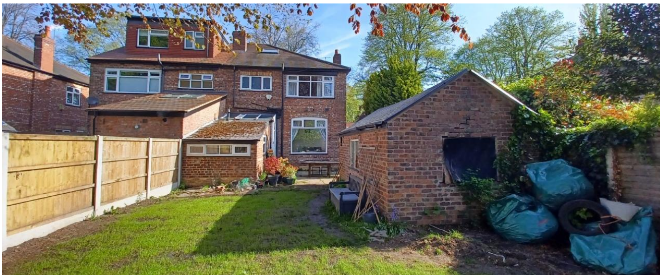
Figure 3. Rear view of property.
