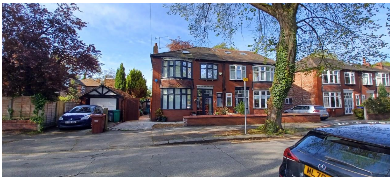
Figure 1. Principal elevation of No.3 Longton Avenue.
