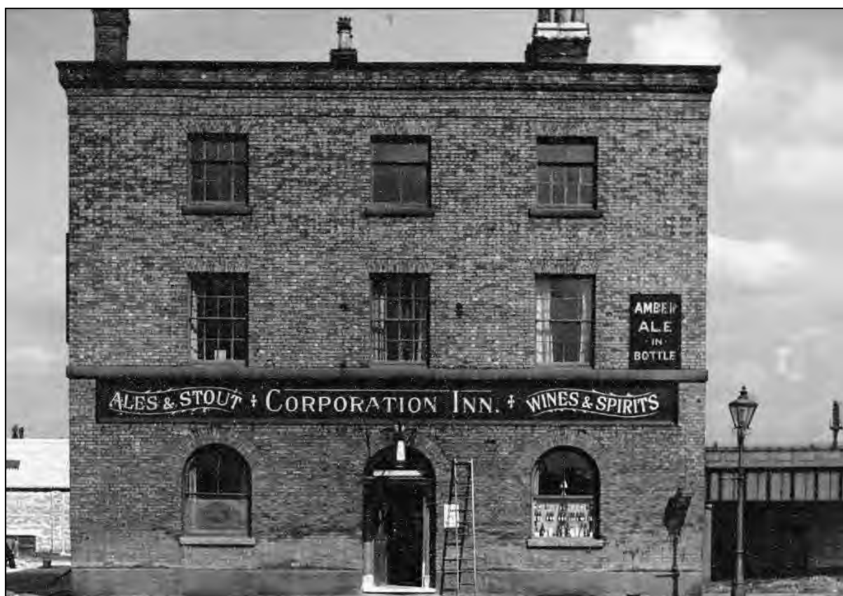
Plate 52: The Cooperation Inn, 1956, with the railway viaduct visible in the background
