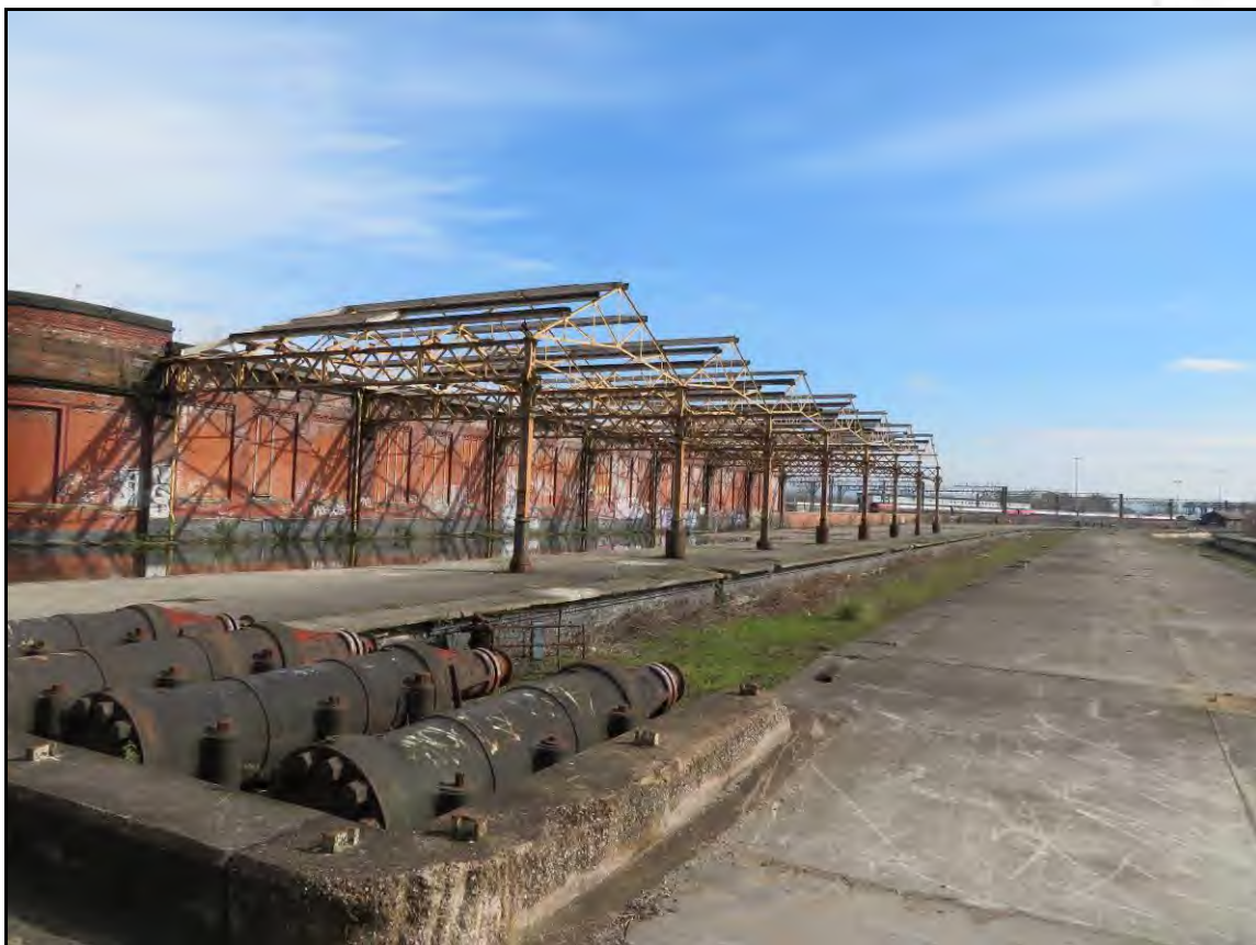
Plate 18: The platforms and hydraulic buffer stops at Mayfield Railway Station, March 2019.
