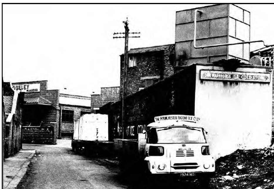
Plate 53: The Mayfield Ice Factory in 1963, with Moseley Plastics in the background
