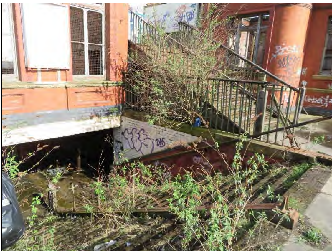
Plate 19: Stairs at Mayfield linking the ground floor to the platforms, March 2019
