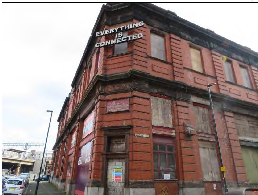
Plate 40: The ticket office at the former Mayfield Railway Station
