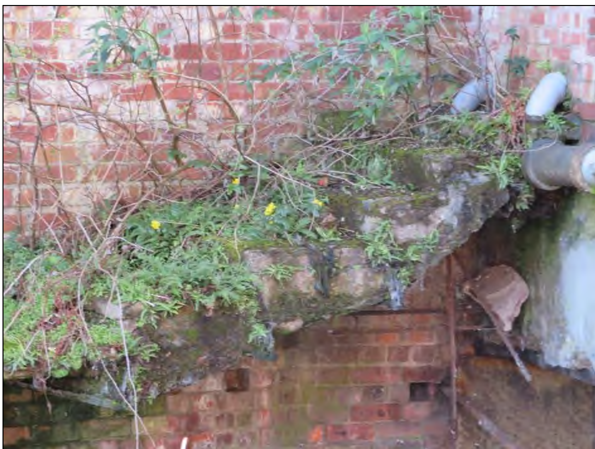
Plate 34: Steps remaining possible from 'Block 2' of the Mayfield Printworks, March 2019
