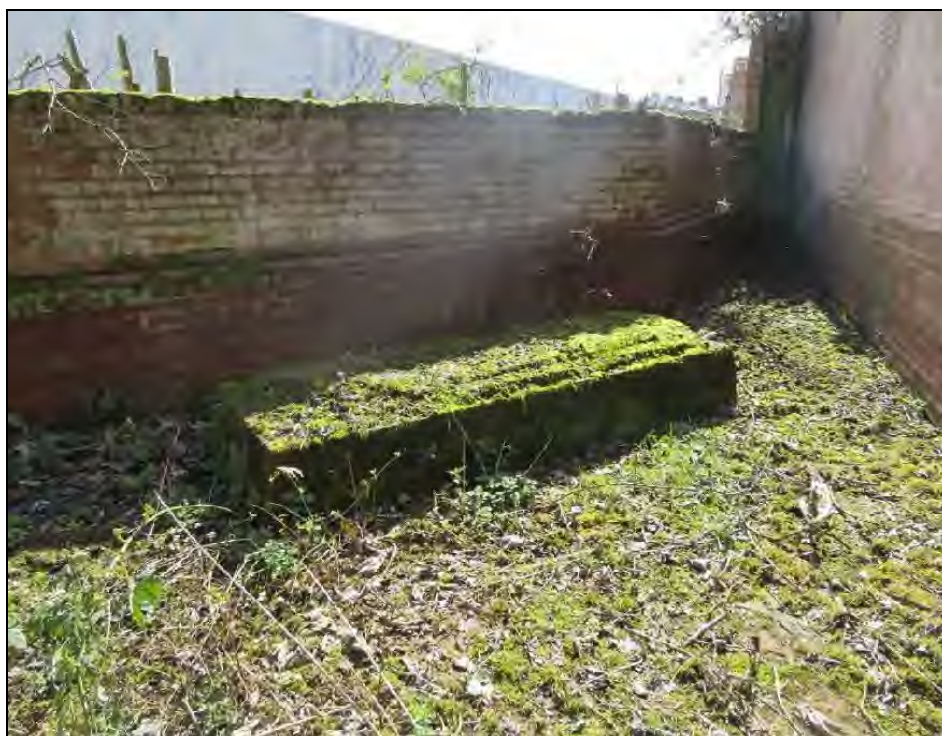
Plate 37: Remaining engine bed within ‘Block 5’ identified on the site visit, March 2019
