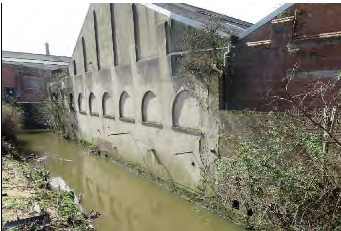
Plate 33: A remnant of the Mayfield Printworks, photographed in March 2019. The apex roof is a modern addition.
