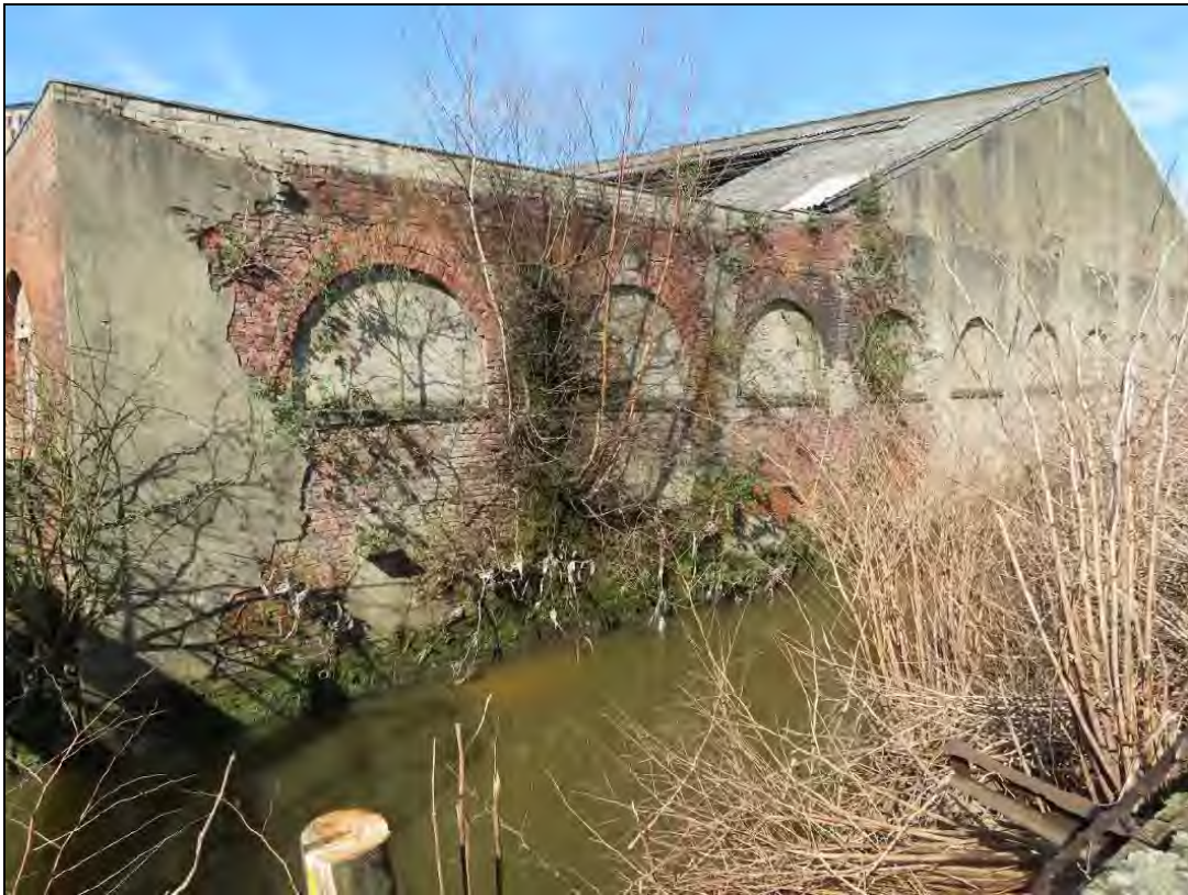
Plate 64: Photograph of the standing remains of the Mayfield Printworks
