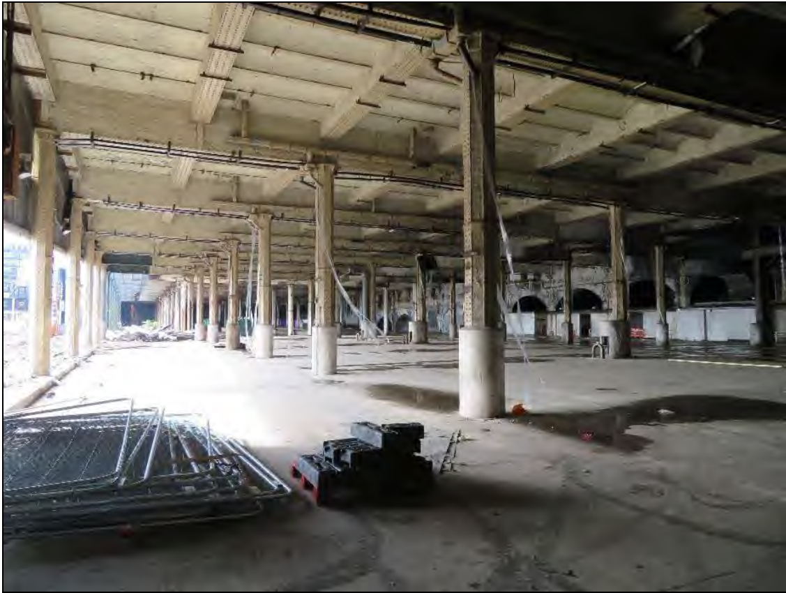
Plate 42: Area beneath the platform at the former Mayfield Railway Station
