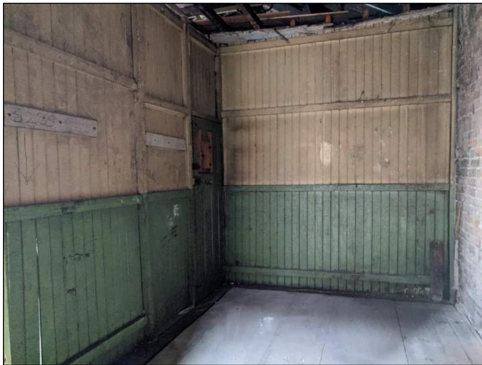
Plate 72: Timber panelling around staircase
