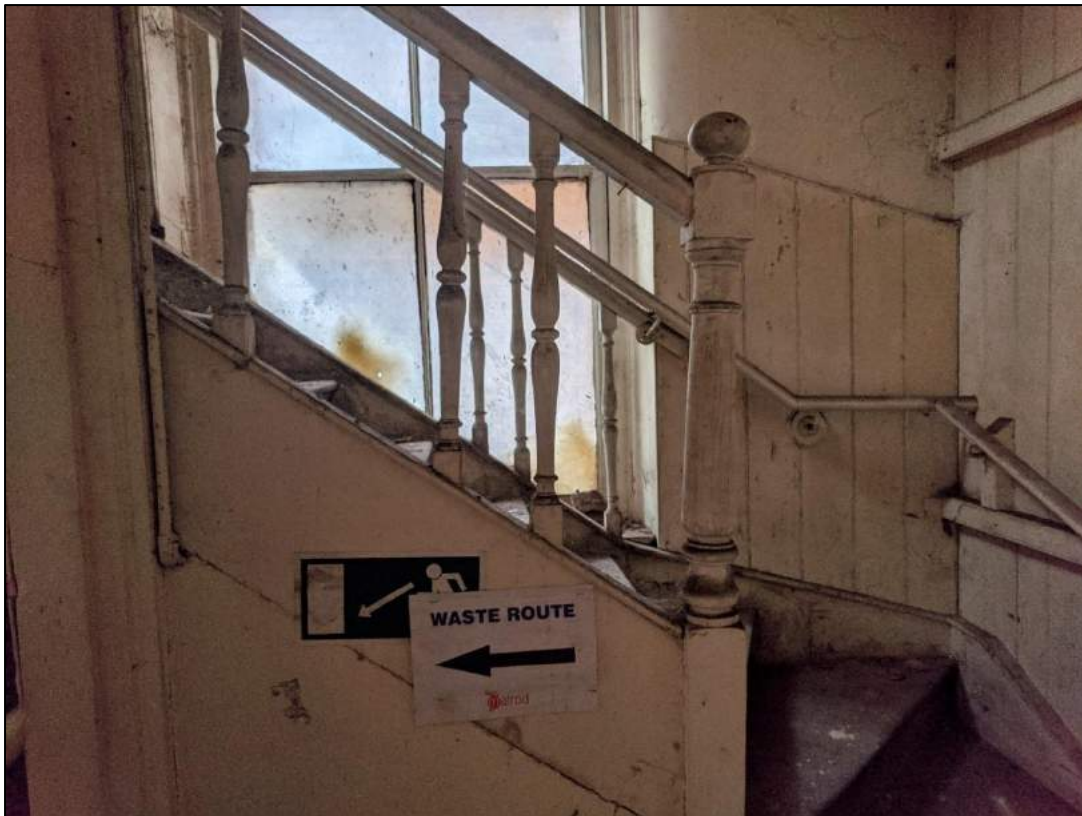
Plate 33: Staircase within extension
