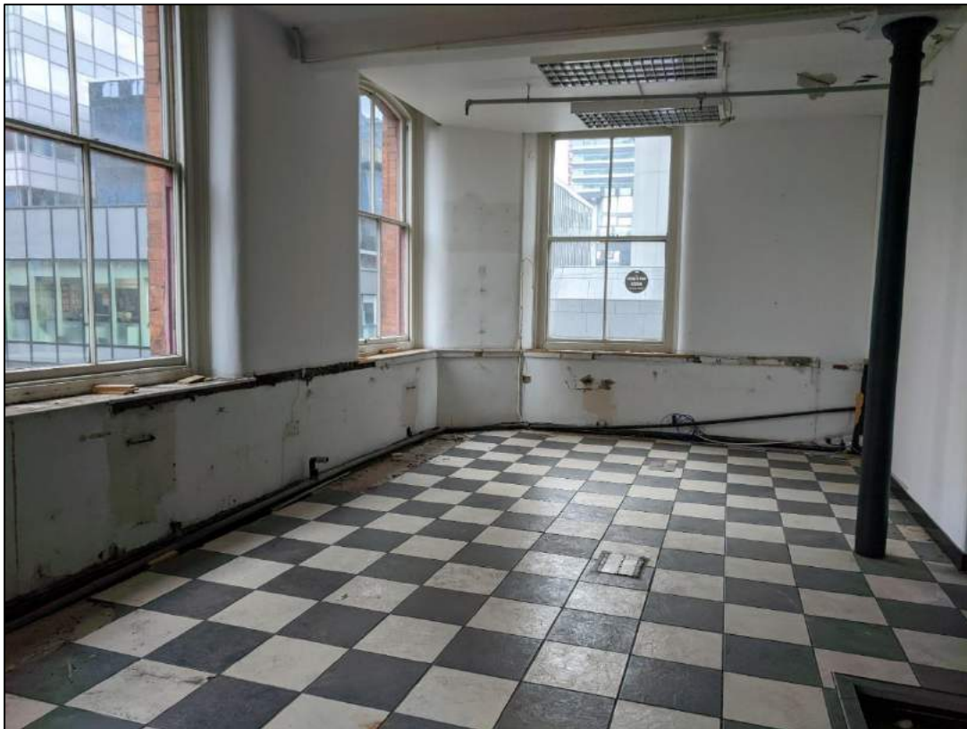
Plate 37: Room to western end of main building
