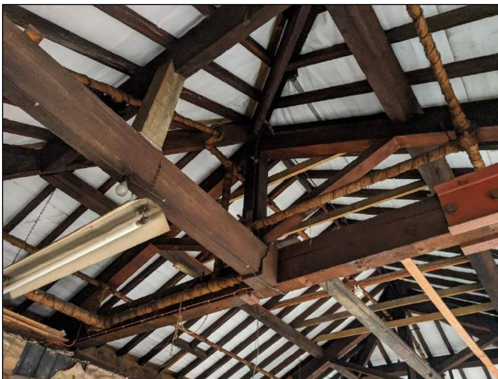
Plate 76: King post truss
