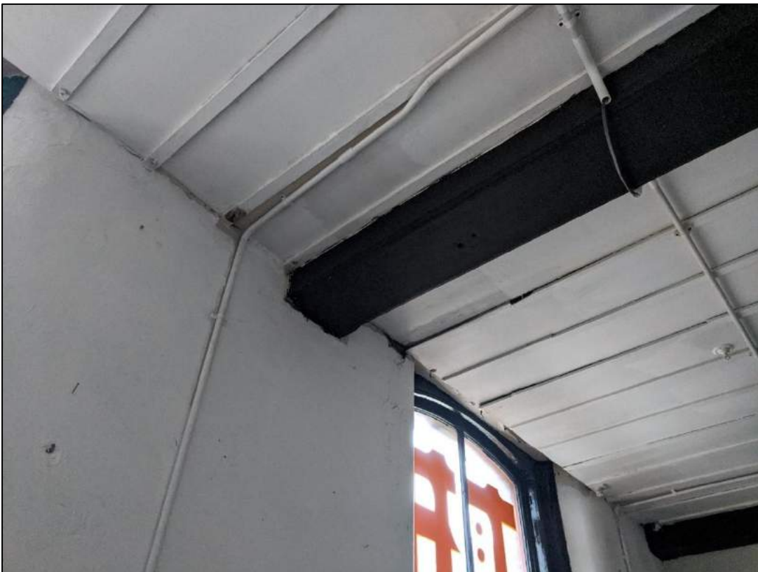
Plate 30: Chamfered and stopped beam
