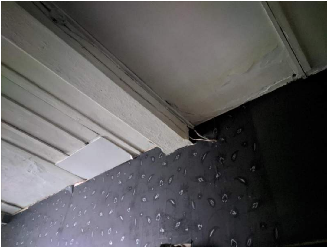
Plate 27: Chamfered and stopped beam
