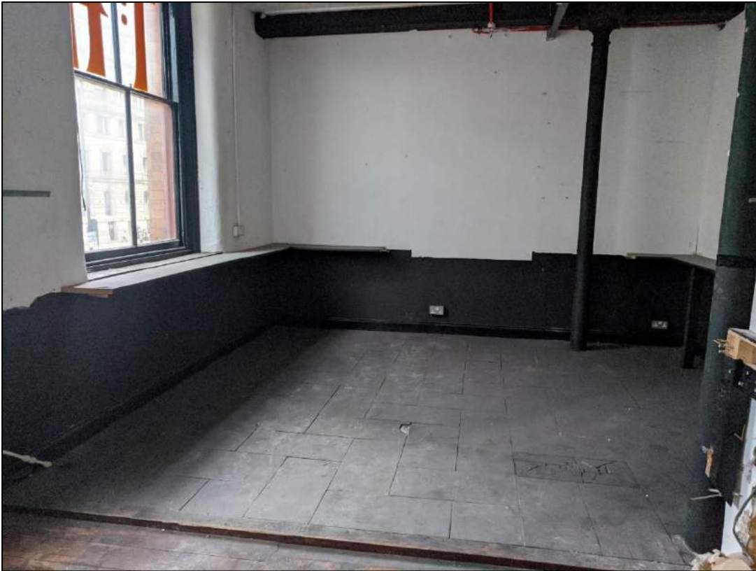
Plate 29: Inserted work space with false floor
