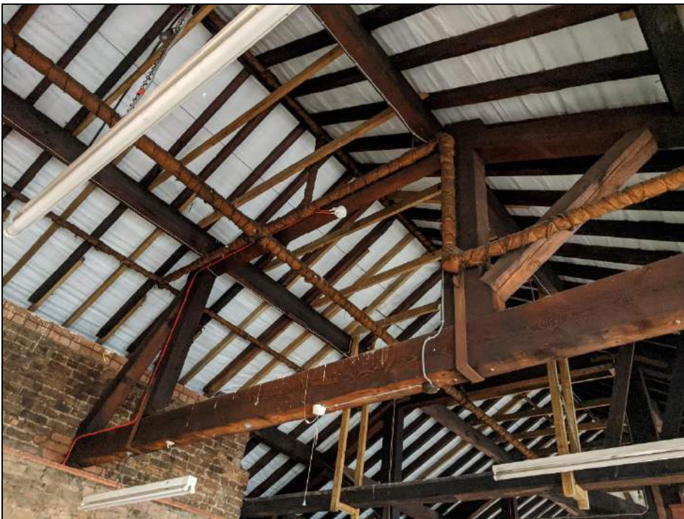
Plate 74: Queen post truss and modern roof
