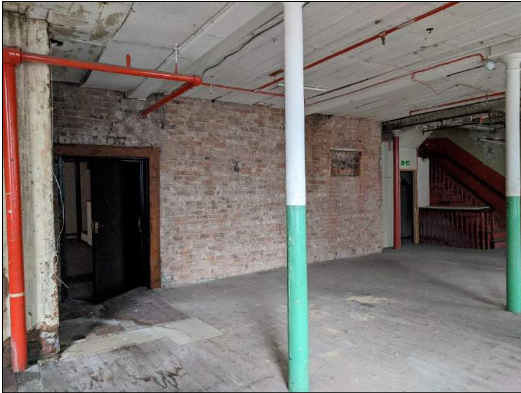
Plate 43: As above looking towards staircase
