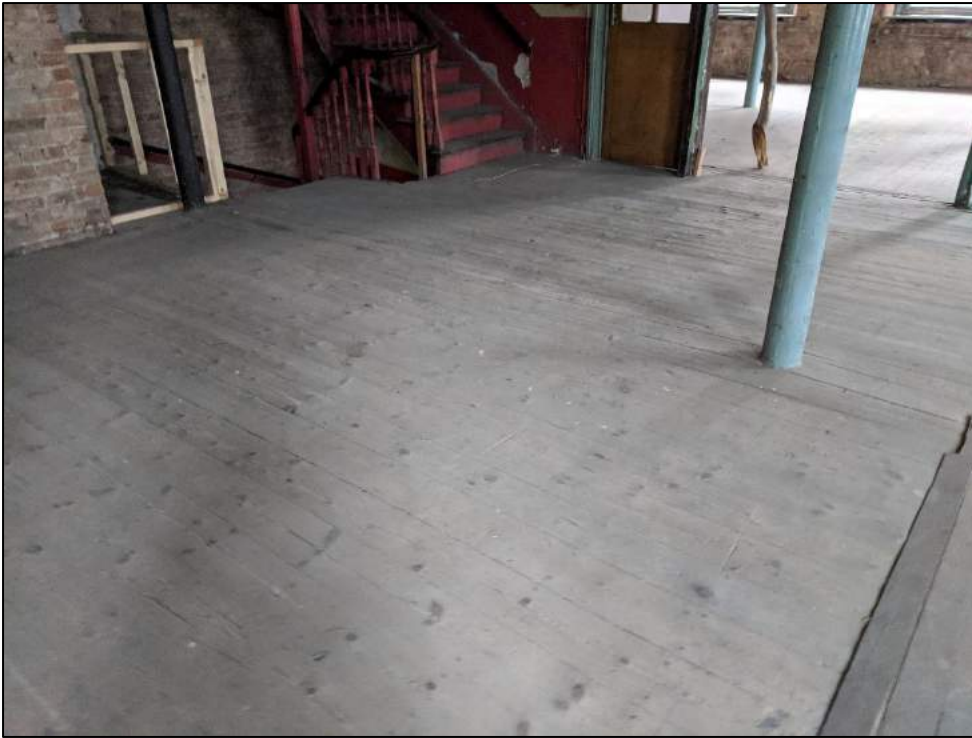
Plate 57: Example of timber floorboards
