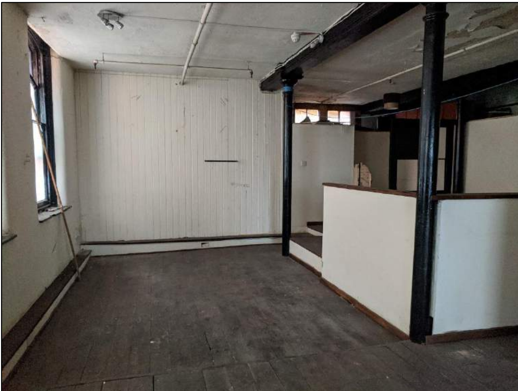
Plate 48: Extension showing inserted walls
