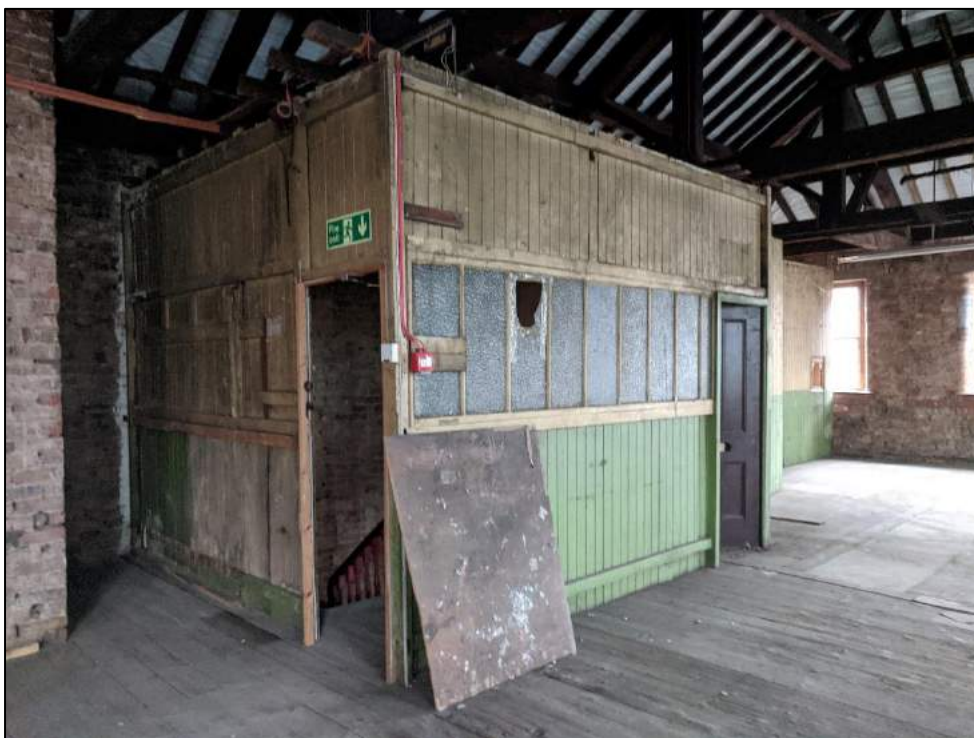
Plate 68: Timber panelling around main staircase
