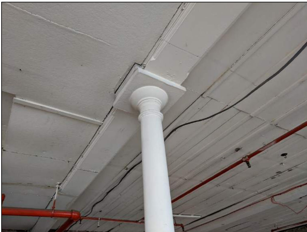
Plate 44: Stanchion capital and beam detail
