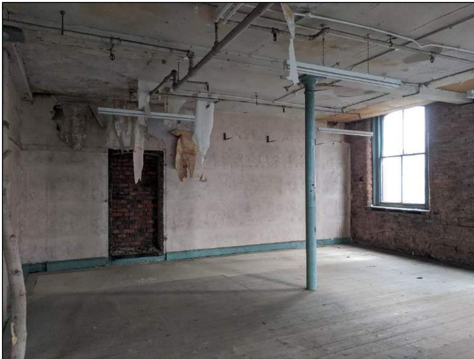
Plate 59: South wall of main building showing inserted and blocked doorway to neighbouring building
