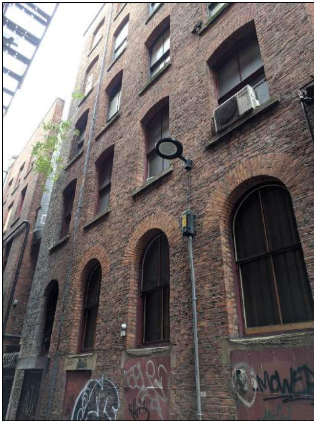
Plate 17: Ground floor of extension
