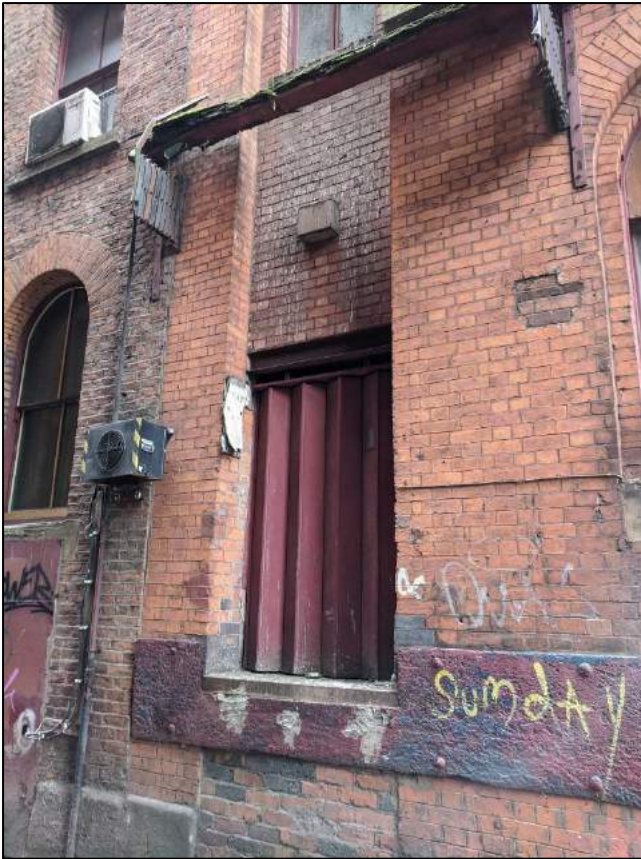
Plate 15: Recessed loading bay with goods lift
