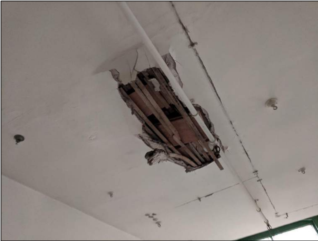
Plate 51: Lath and plaster ceiling
