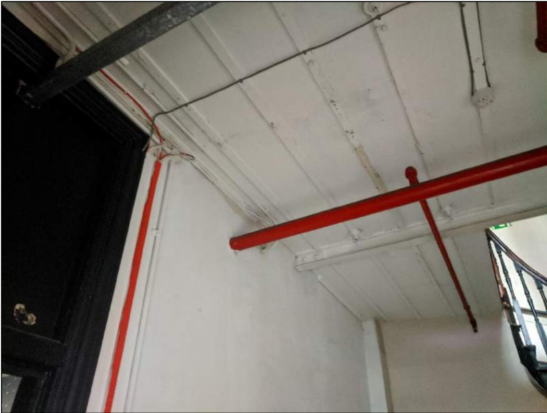
Plate 25: Timber ceiling detail
