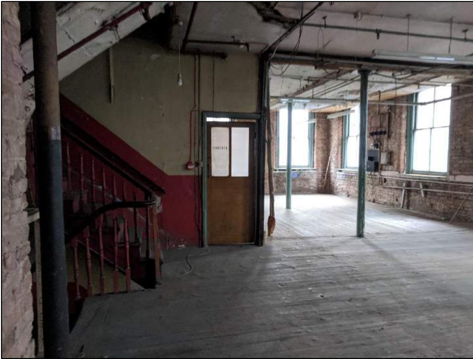
Plate 55: As above looking towards the west side
