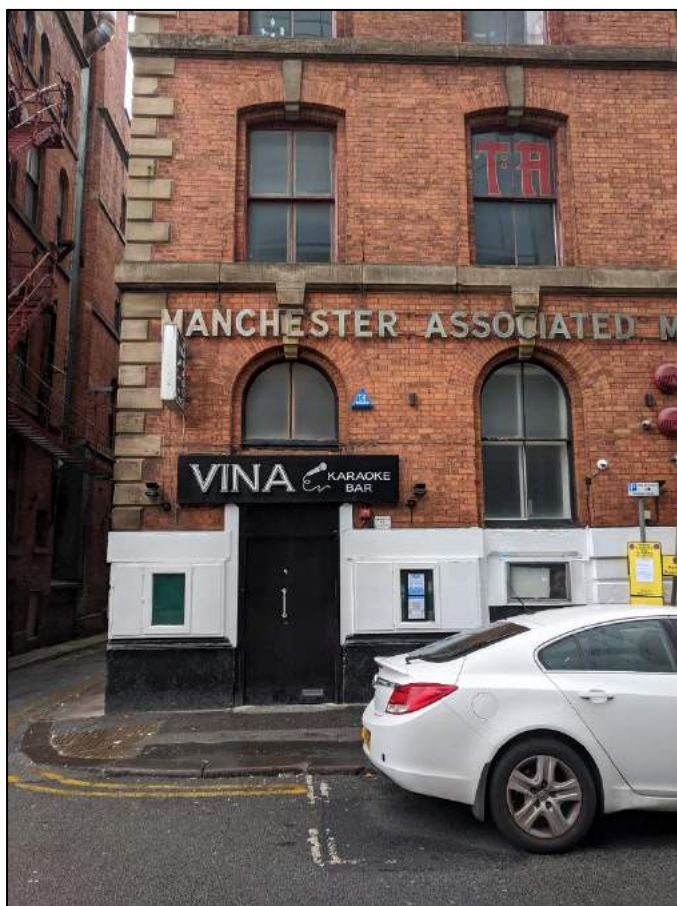
Plate 4: Inserted doorway at eastern end
