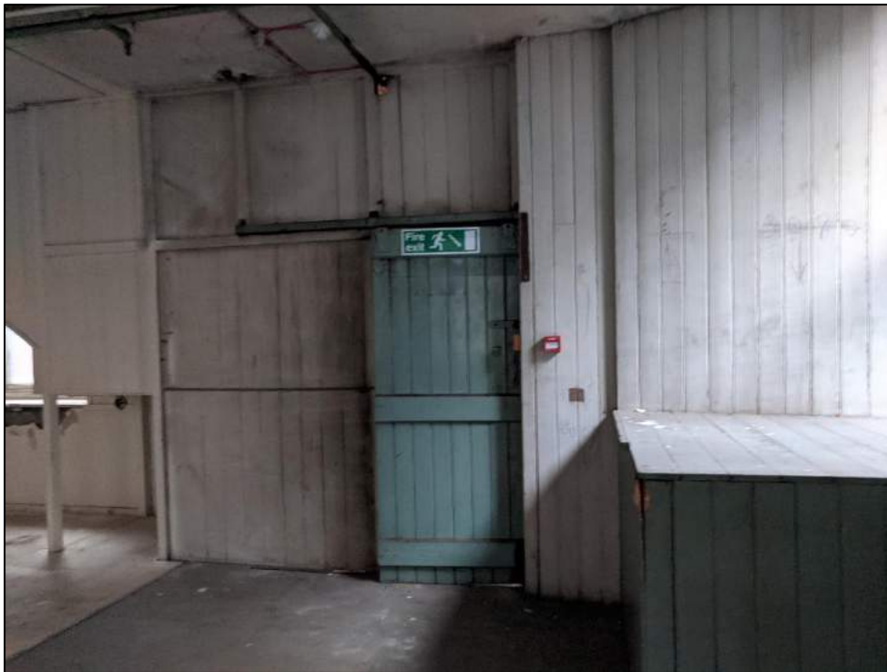
Plate 63: Timber panelling hiding staircase within extension
