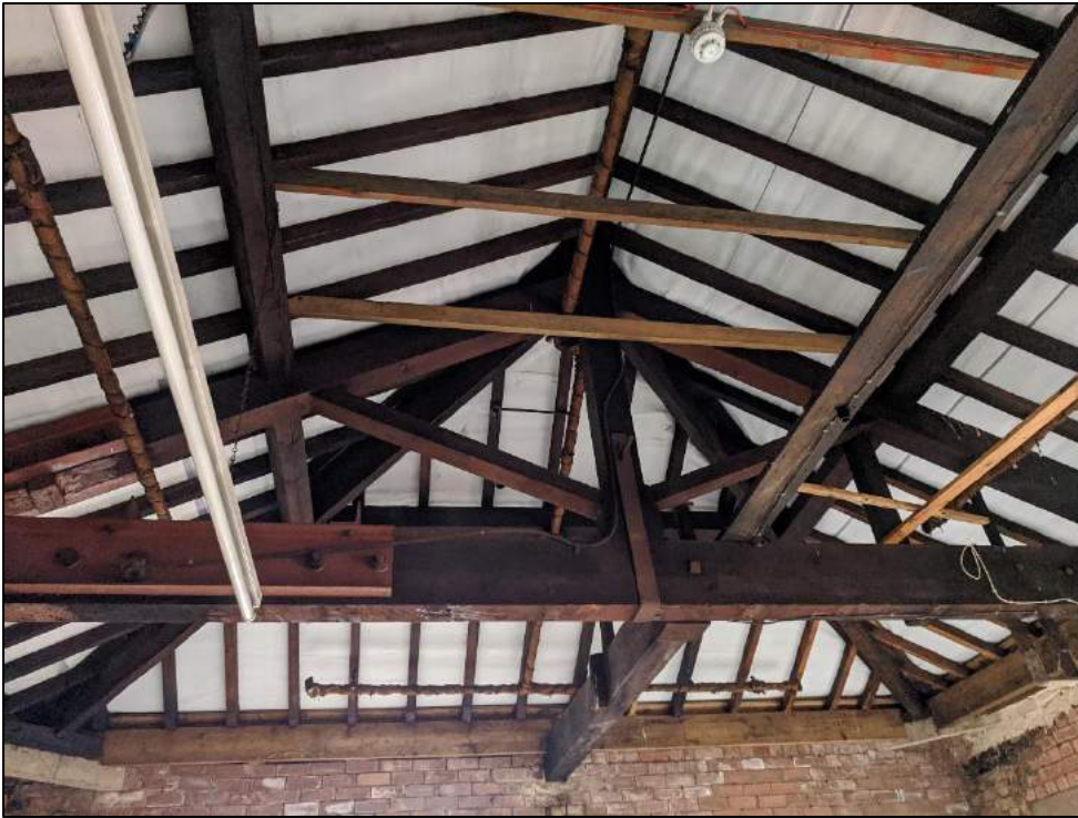
Plate 77: King post truss
