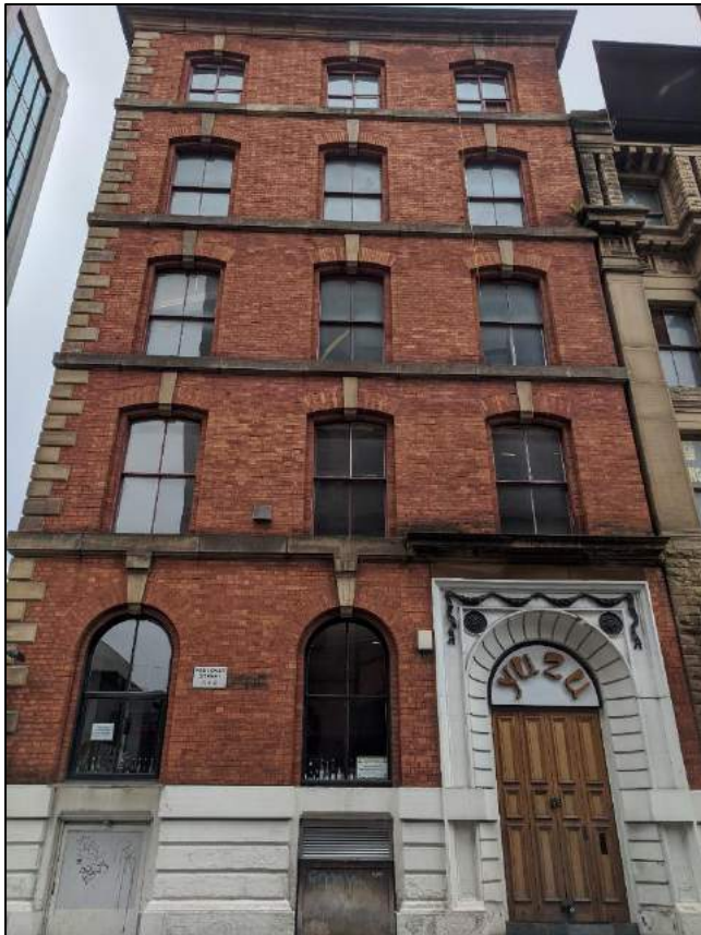
Plate 8: West elevation to Faulkner Street
