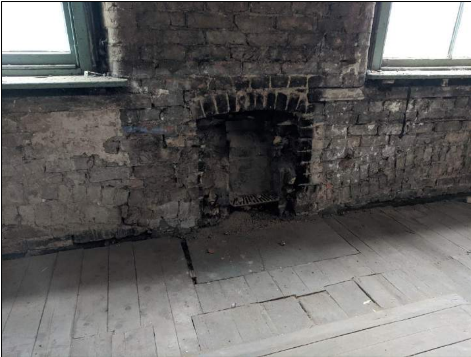
Plate 61: Fireplace in northern wall
