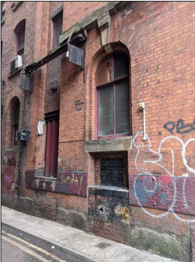
Plate 14: As above showing window detail
