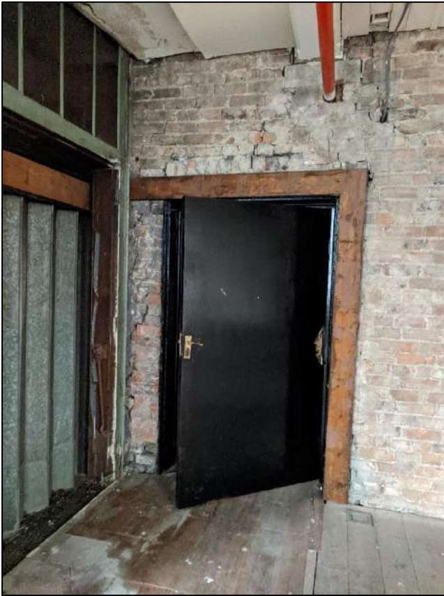
Plate 45: Inserted doorway into extension
