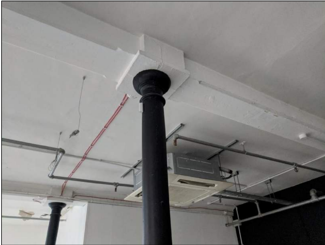
Plate 39: Stanchion capital in main building with chamfered and stopped beam
