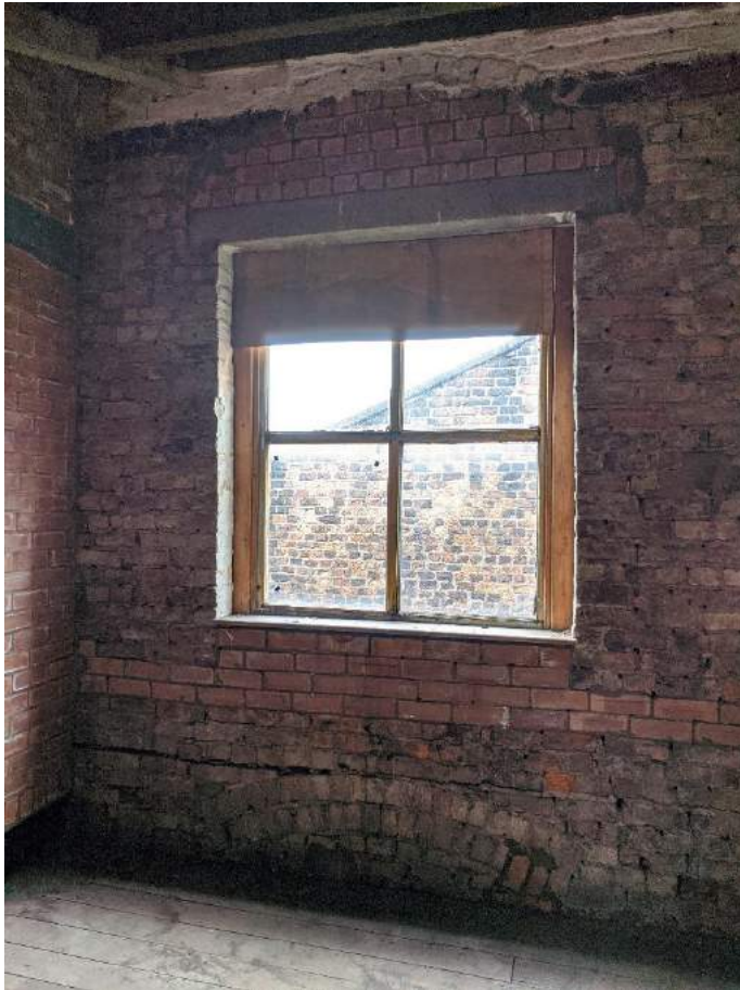
Plate 71: Window detail showing concrete lintel
