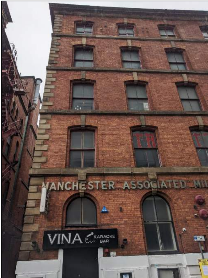
Plate 5: Upper floors at eastern end
