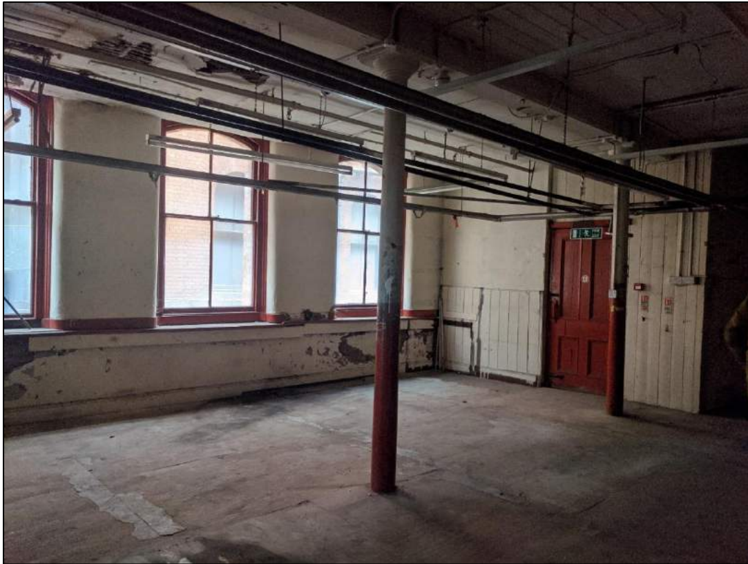
Plate 31: Extension showing cast iron stanchion and doorway to staircase
