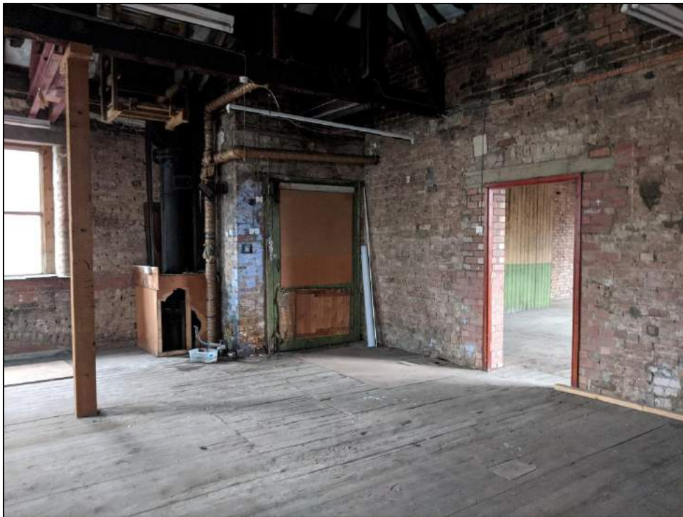
Plate 67: Goods lift and inserted entrance to extension
