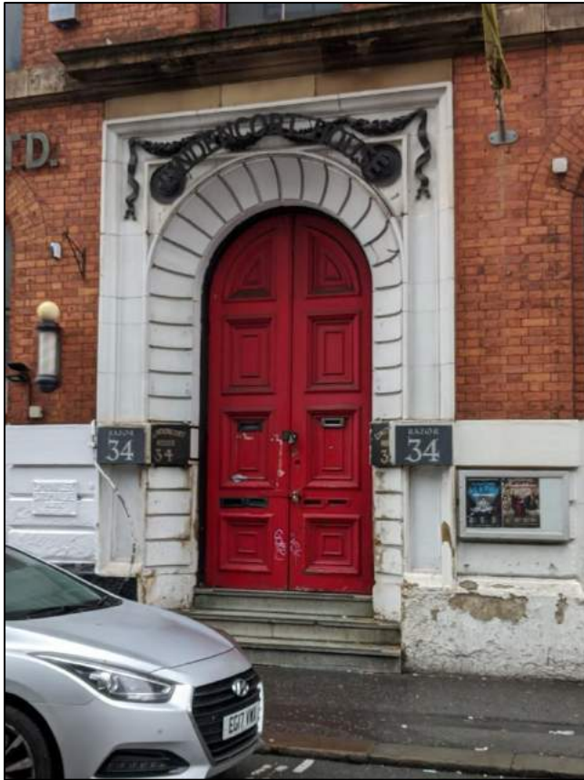
Plate 7: Main entrance to bay 4
