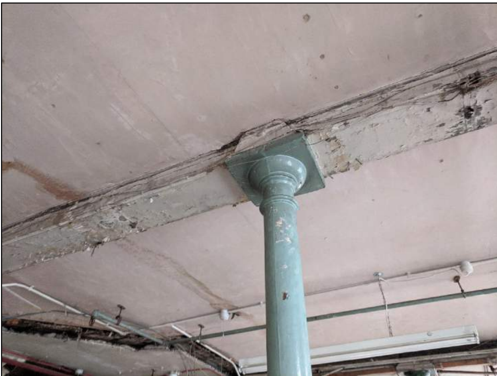
Plate 58: Stanchion capital and timber beam
