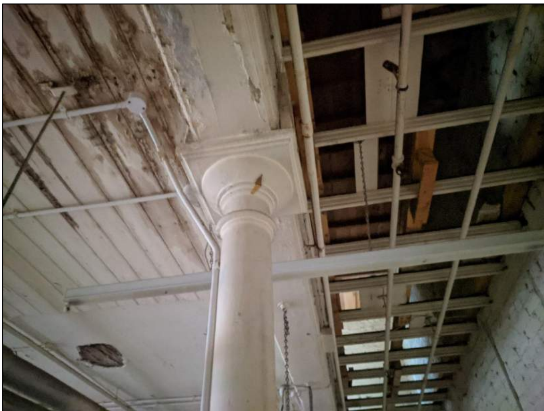
Plate 32: Stanchion capital with remains of former light well (right)
