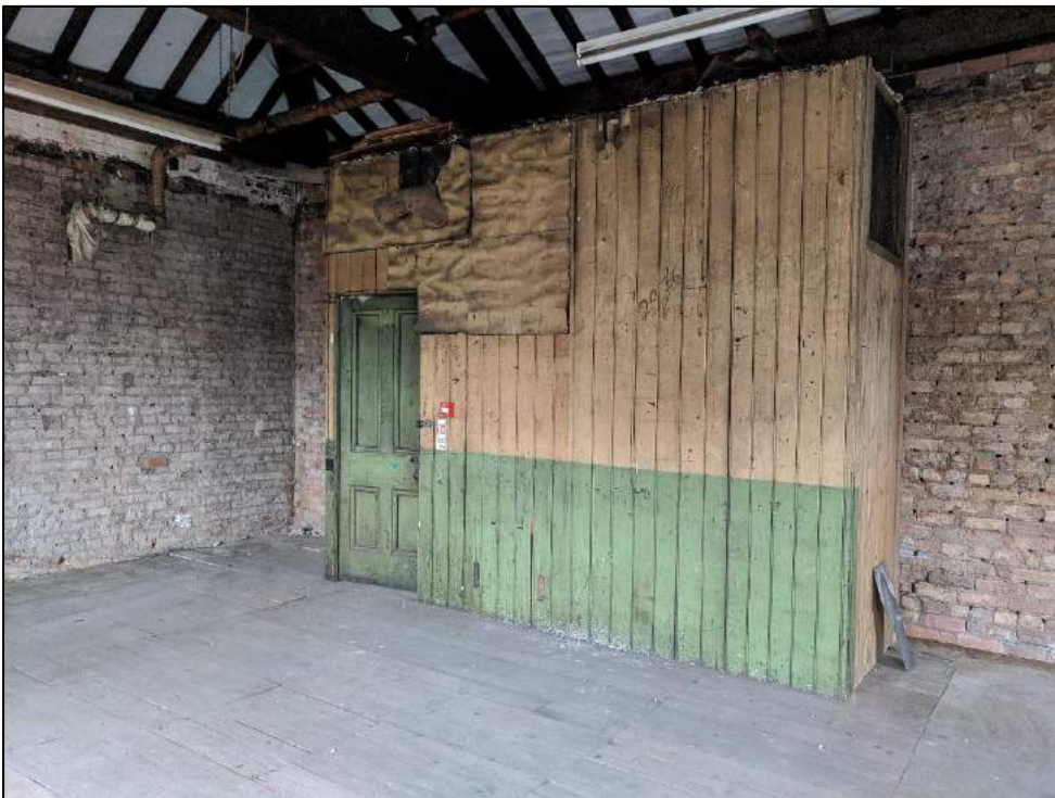
Plate 78: Timber panelling containing extension staircase
