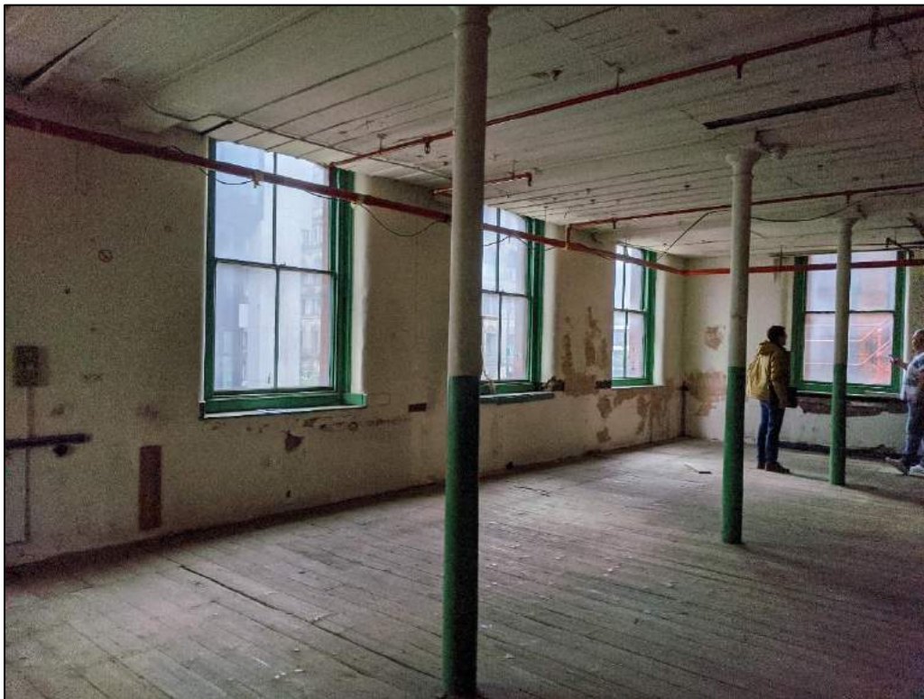
Plate 40: Second floor of main building
