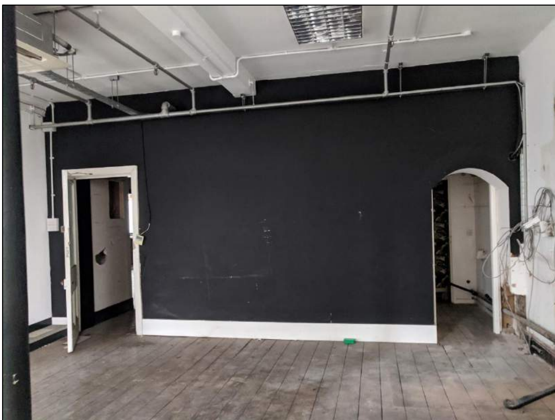
Plate 38: Inserted wall
