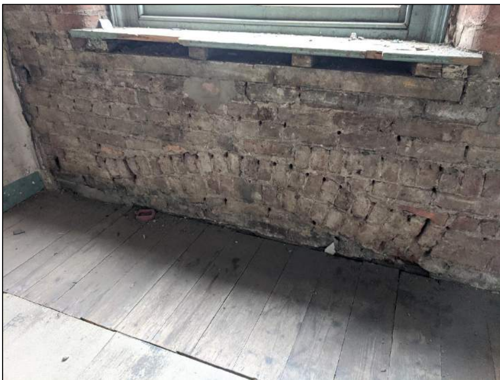
Plate 60: Detail of walling showing brick arch of window below
