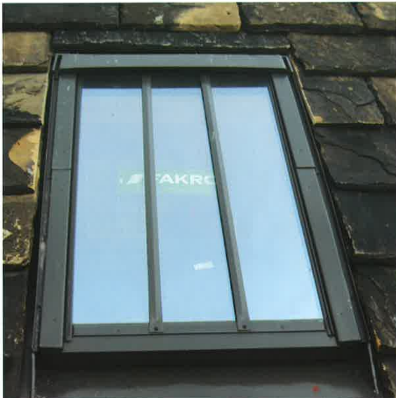
Conservation window with two mullion bars
