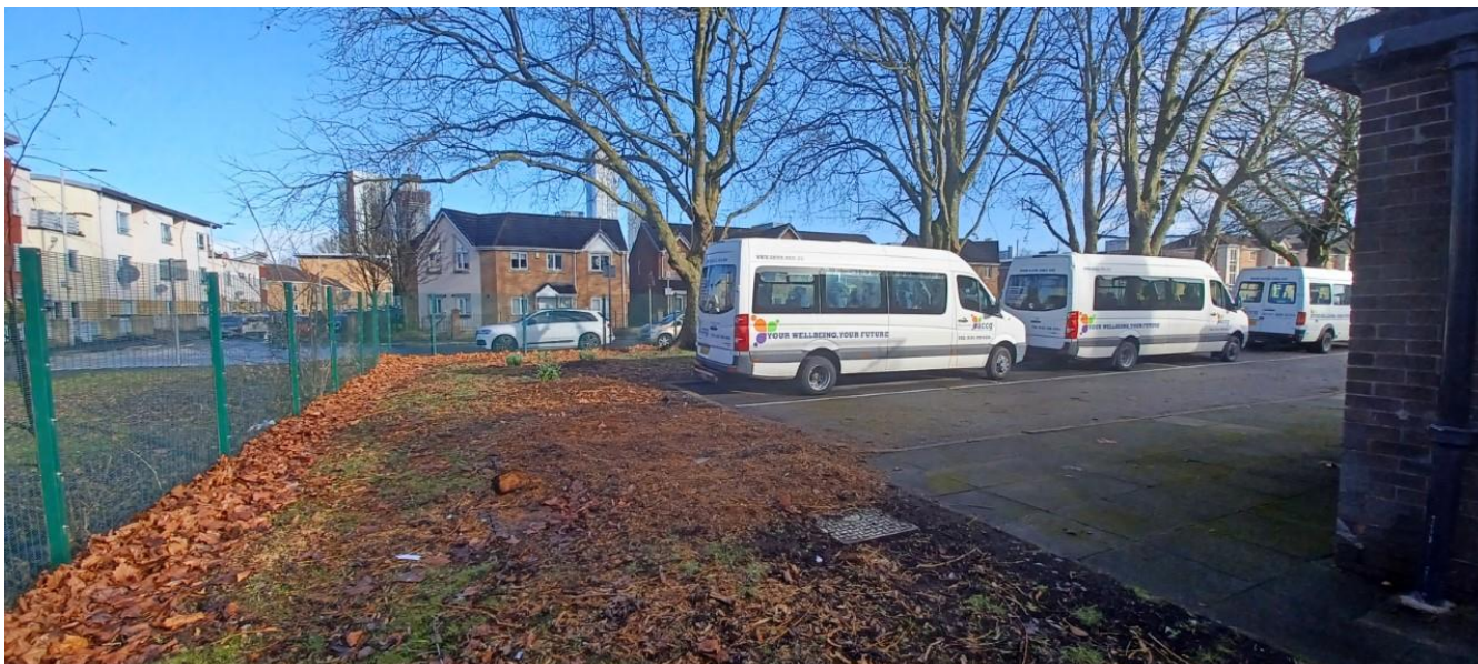
Figure 2. Proposed site of air source heat pumps.
