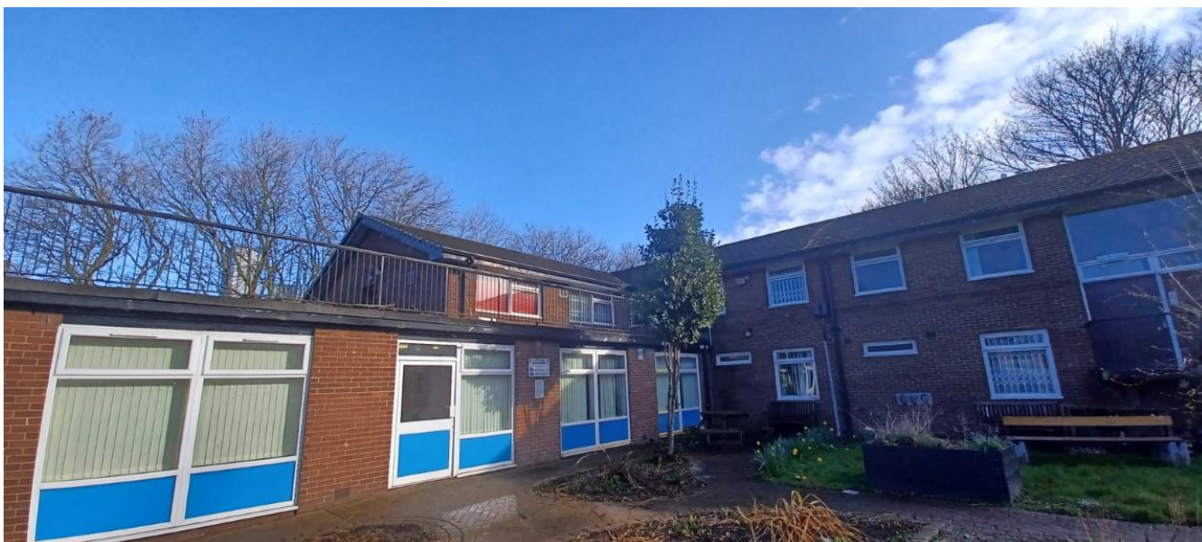
Figure 3. Proposed site of photovoltaic panels.
