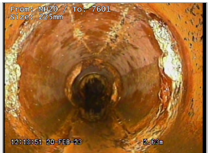
Attached deposits, encrustation from 12 to 12 o'clock 10% cross-sectional area loss, Start
