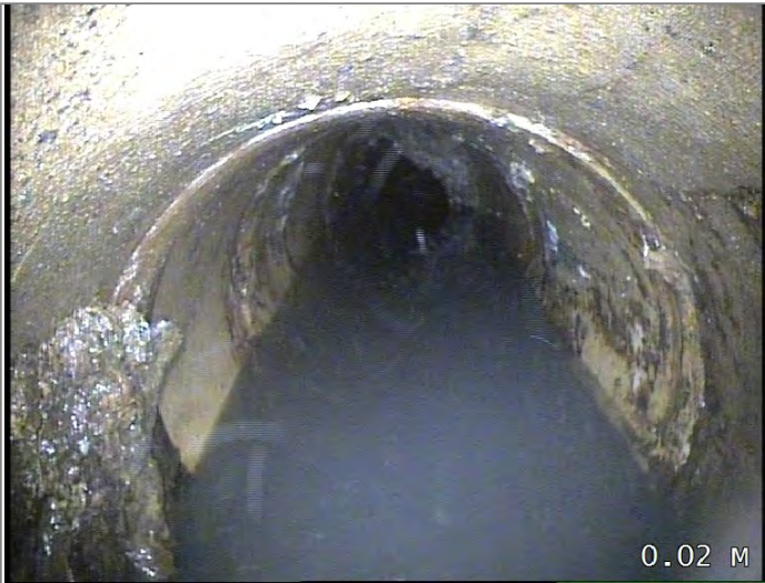
Start node type, manhole, reference MH07A
