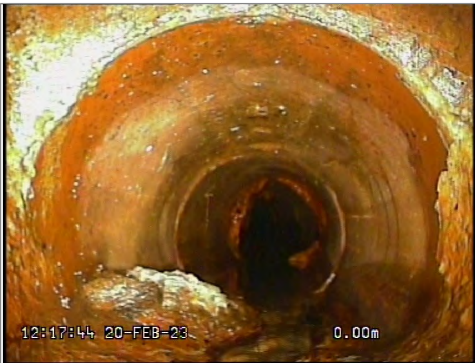
Start node type, manhole, reference MH20
