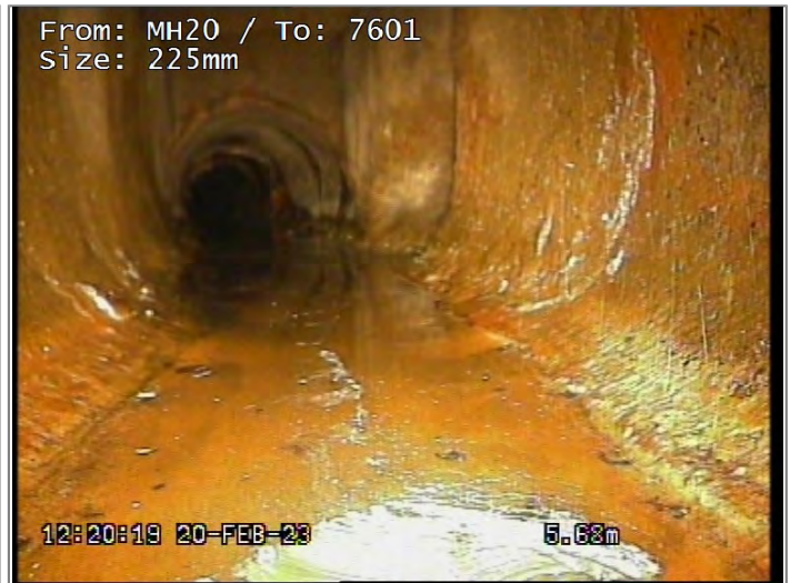
Attached deposits, encrustation from 12 to 12 o'clock 10% cross-sectional area loss, Finished
