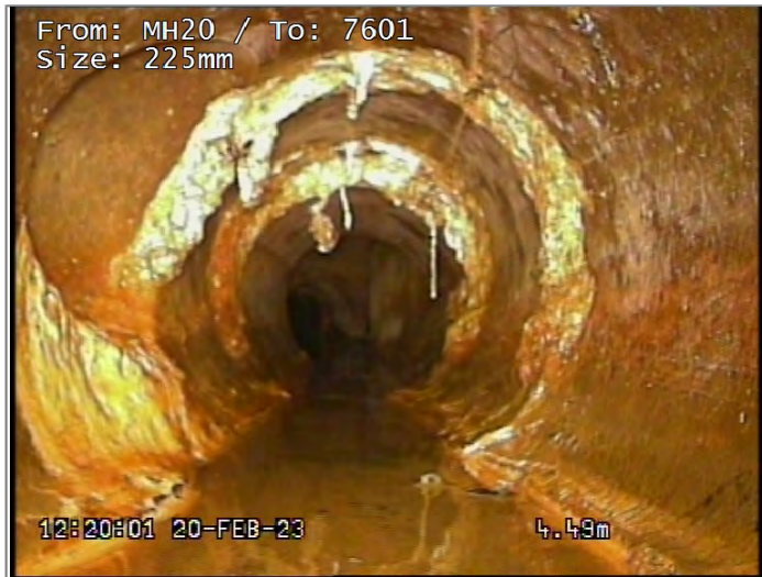
Junction at 10 o'clock, diameter 150mm
