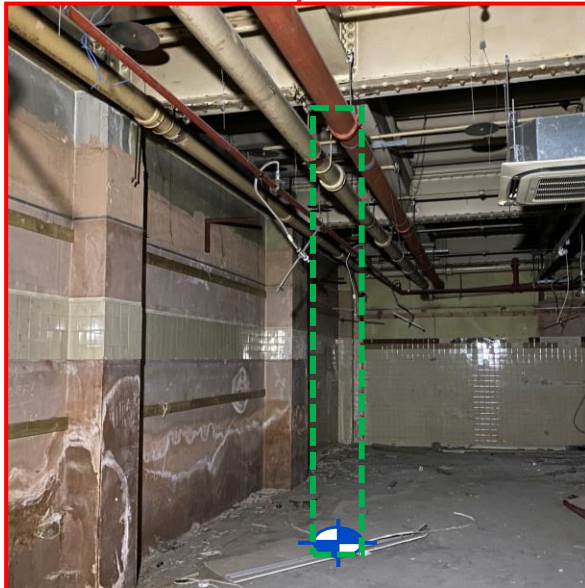
Picture of the location at B1
