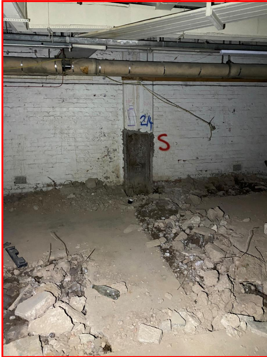
Picture of existing basement slab penetration.
