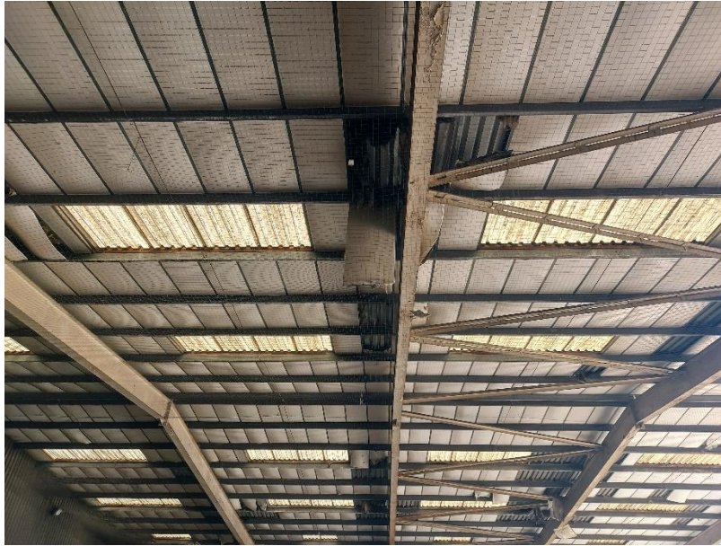
PLATE 7 SHOWING INTERNAL BIRD NETTING
