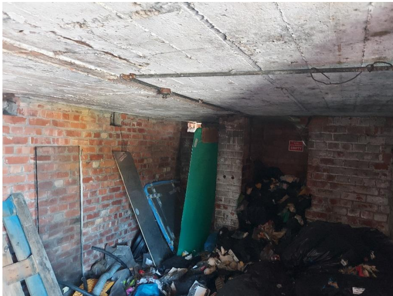
PLATE 11 SHOWING BUILDING INTERNALS
