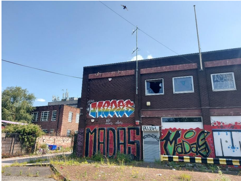
PLATE 1 SHOWING SOUTH WEST FACING ASPECT OF B1a
