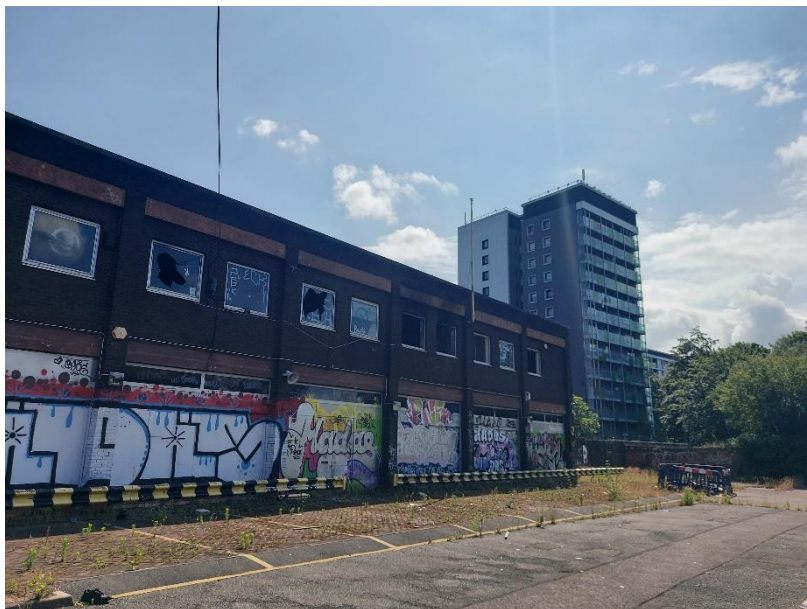
PLATE 2 SHOWING SOUTH WEST FACING ASPECT OF B1a
