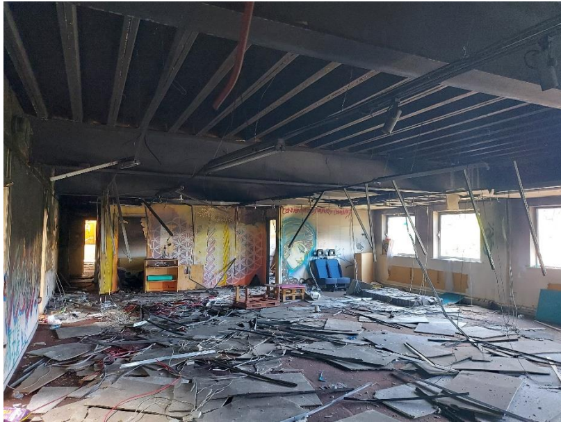
PLATE 5 SHOWING THE INTERNAL OF BUILDING B1A
