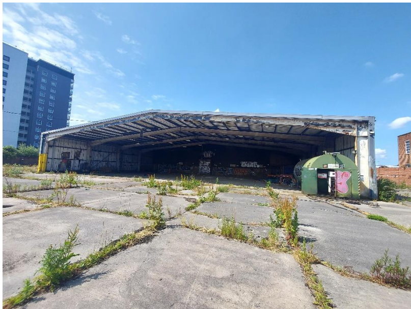
PLATE 6 SHOWING NORTH-EAST FACING ASPECT
