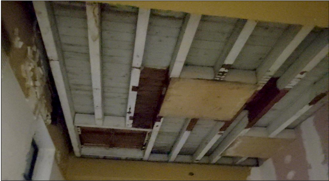
Photograph of the exposed timber flooring within the proposed WC/storage area.
