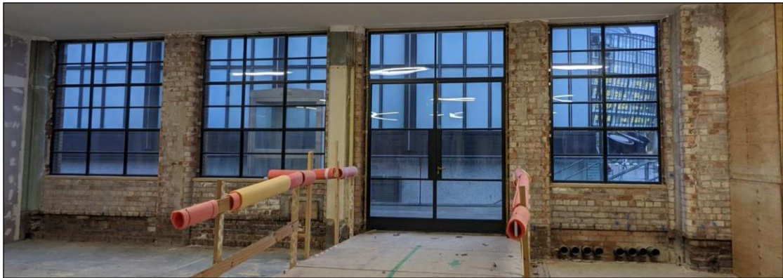
Existing Mayes Street façade, Main Entrance (to be retained)
