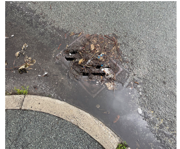
FIGURE 7: BLOCKED DRAIN & PONDING
