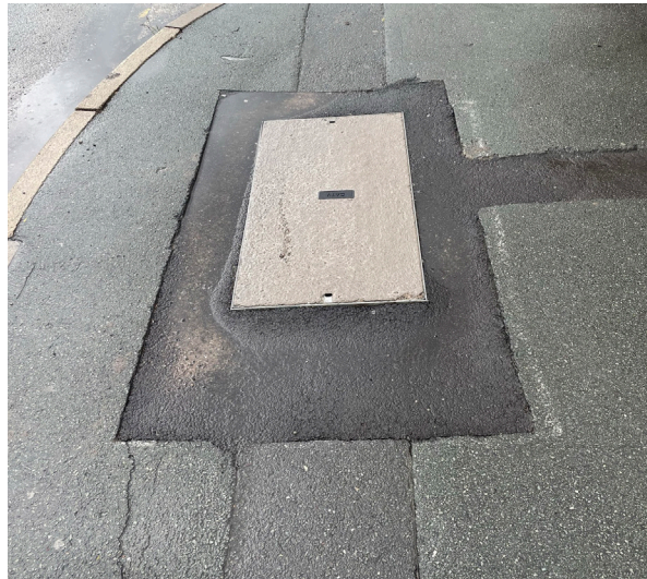
FIGURE 4: SUBSIDENCE GROUND UTILITY CONNECTIONS
