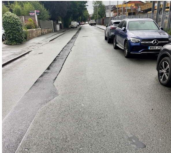
FIGURE 8: ROAD EAST FACING
