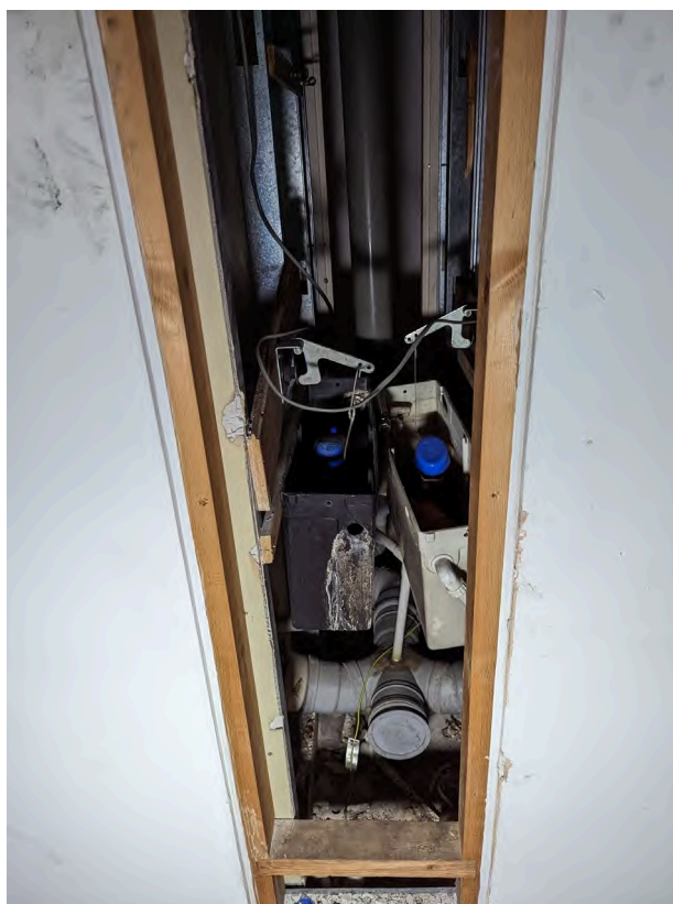
Image 4: Example of pipework associated with former site use
