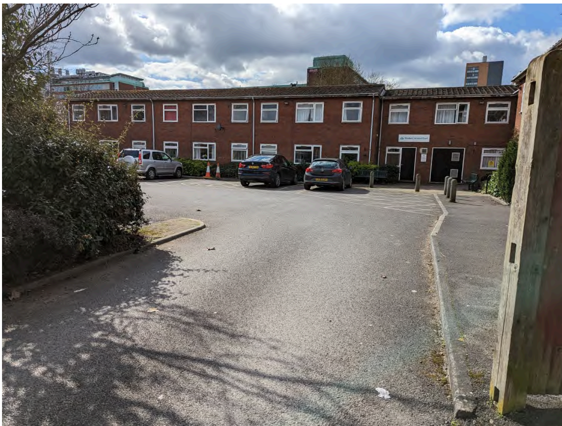
Image 10: Access and hardstanding/carpark for Elizabeth Yarwood Court
