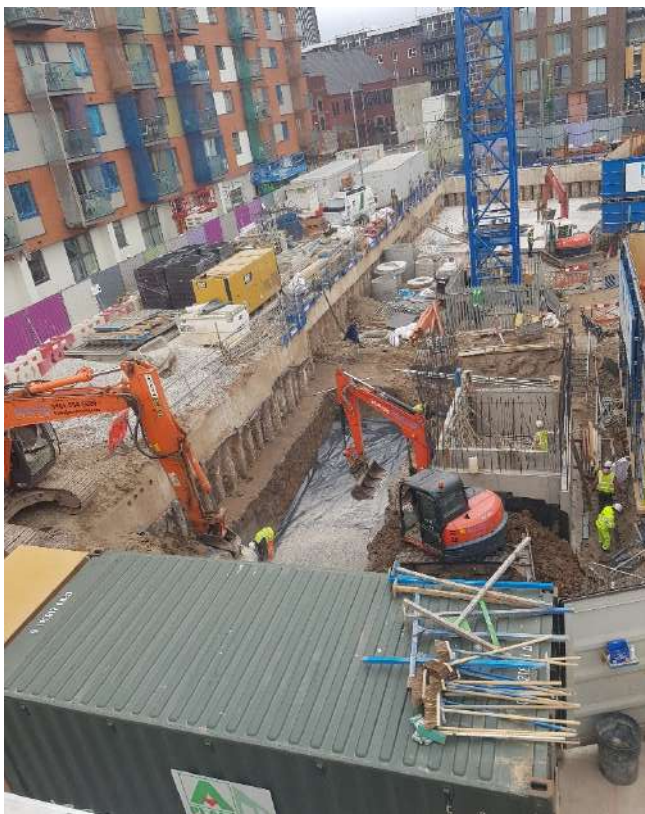
Photo 4 - Attenuation Tank Installation
