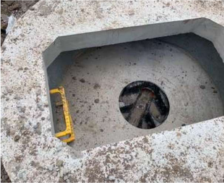
Photo 1 – As built Chamber SW02 Access Point
