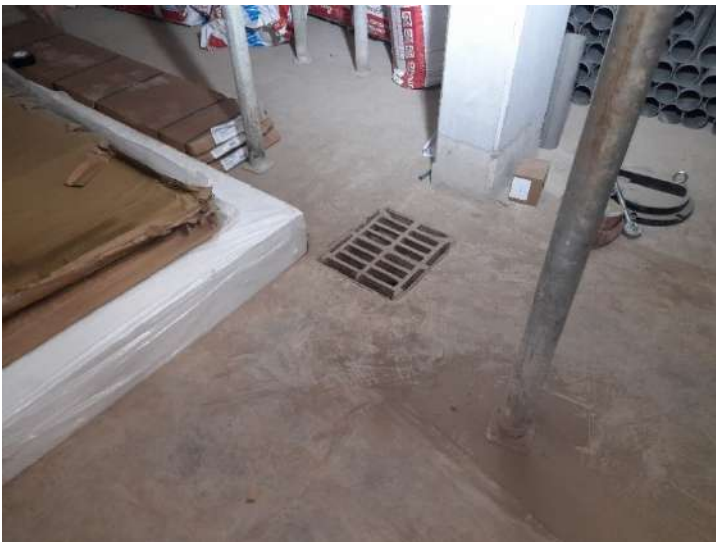
Photo 11 – Surface Water Gully
