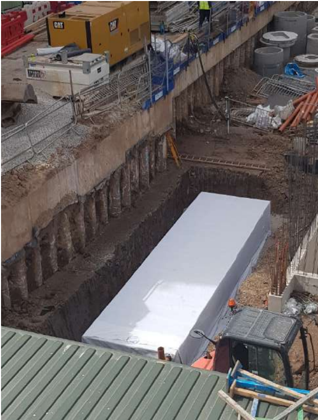
Photo 5 - Attenuation Tank Installation
