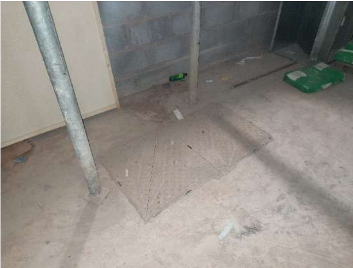
Photo 7 – SW07 Catchpit Cover
