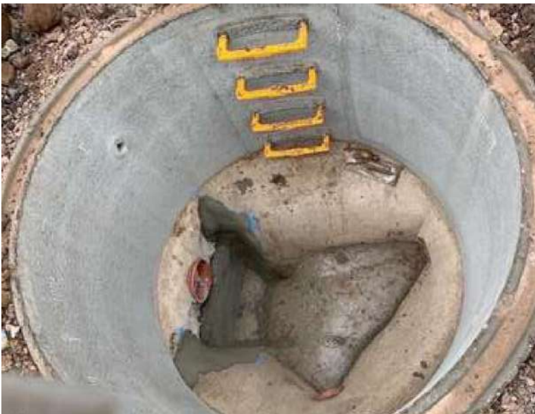
Photo 2 – Chambers SW7 and SW9 either side of the attenuation tanks are in place and being benched up
