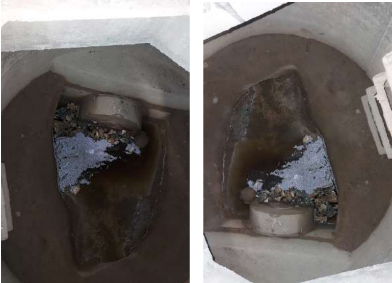
Photo 19 - Flow control manhole
