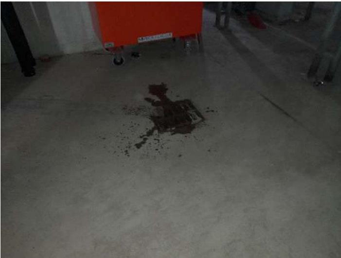
Photo 14 – Surface Water Gully
