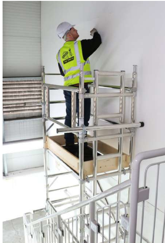
• Illustration 15 – Mobile Scaffold Tower
