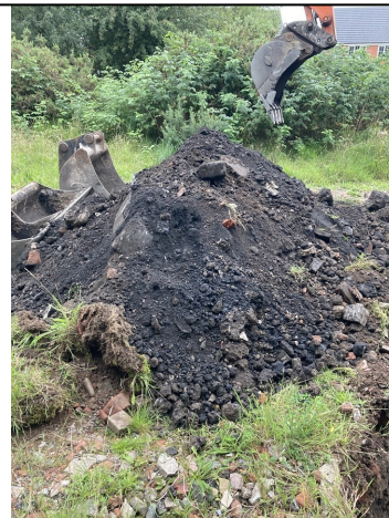
Trial Pit 107 Spoil
