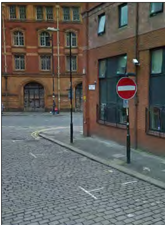
Photo plate 4. Back Acton Street eastern footway. Adequate width and surfacing. Pinchpoints created by street furniture.
