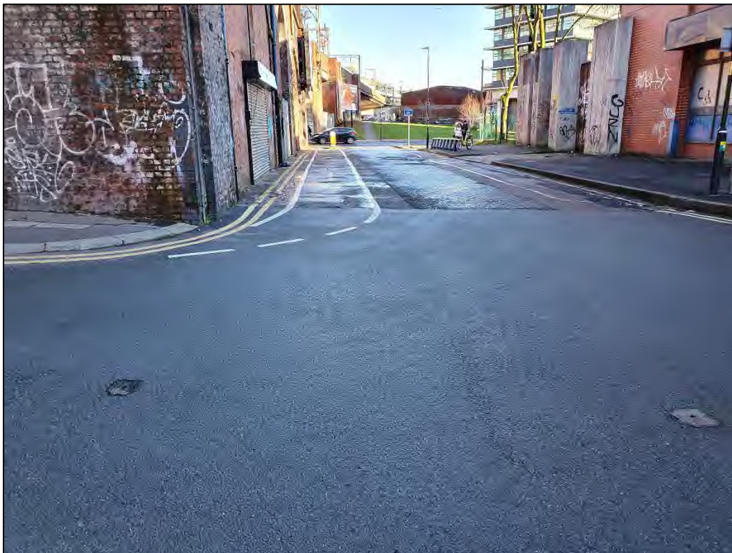
Photo plate 6. Altrincham Street. Southern footway wide with adequate surfacing.
