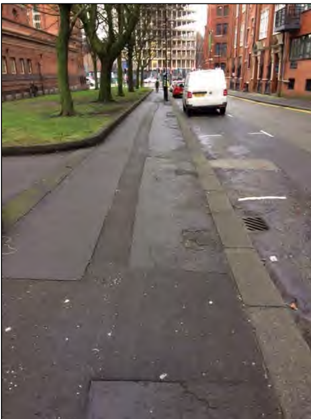
Photo plate 2. Cobourg Street western footway. Generally wide footway with adequate surfacing.
