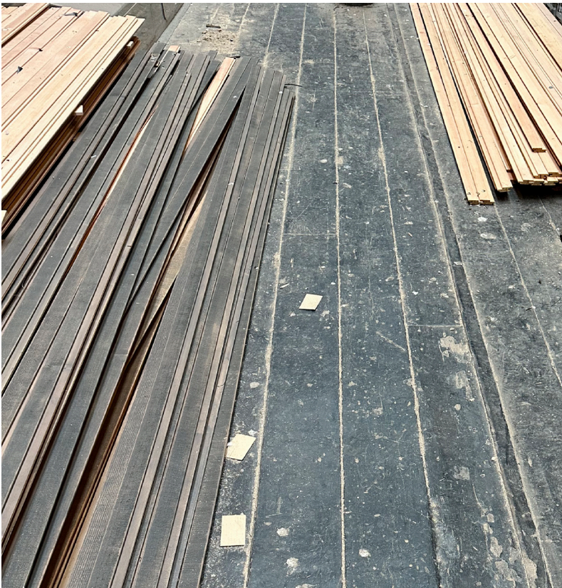
West Platform Historic Floorboards
