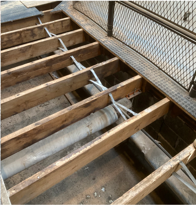
East Platform Sub Structure
