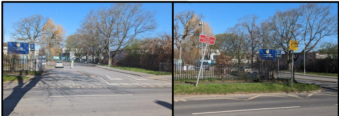
Picture 3-2 and Picture 3-3 – School Keep Clear Markings on Greenbrow Road
