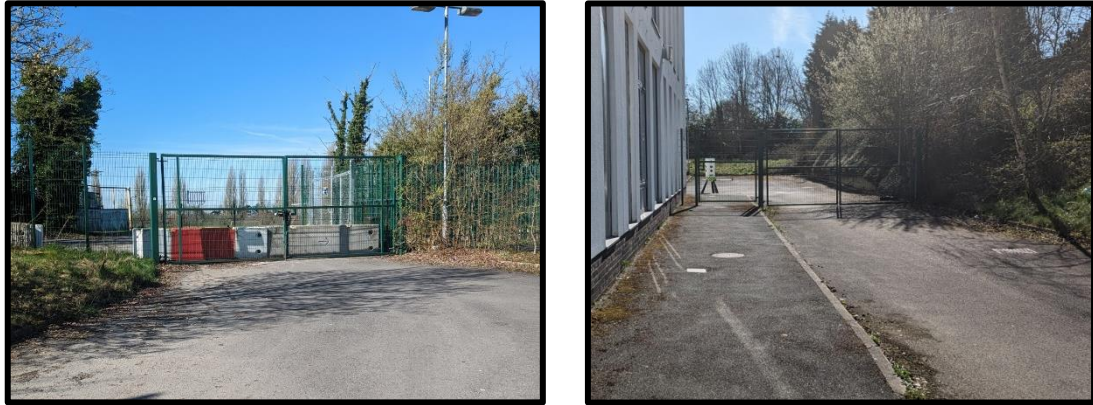
Picture 3-19 and Picture 3-20 – Manual Vehicle Access Gates Outside the Secure Line of the School Site
