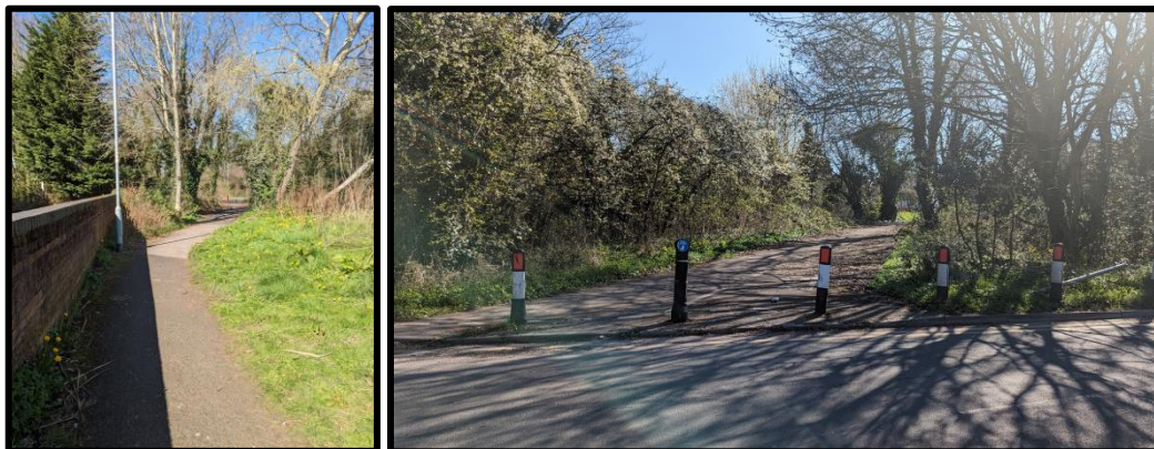
Picture 3-33 and Picture 3-34 – Shared Footway and Cycleway from Capenhurst Close to Clay Lane
