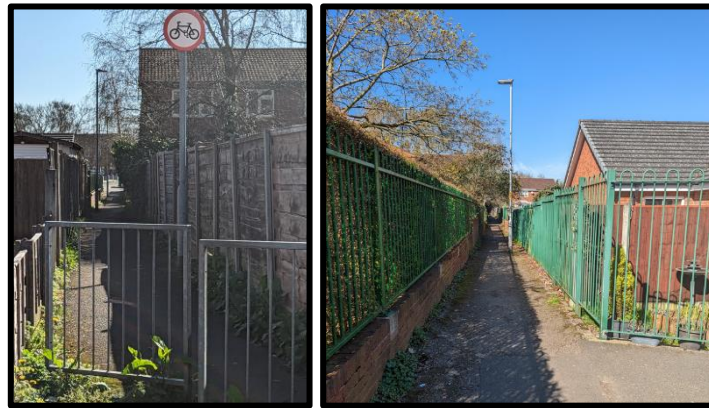
Picture 3-30 and Picture 3-31 – Footpath from Capenhurst Close to Scout Drive
