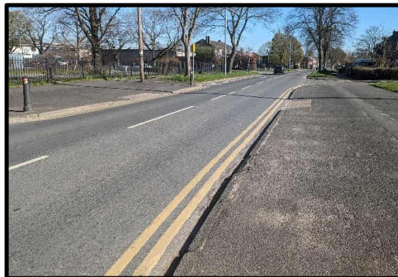
Picture 3-5 – Footway Build-Out at Uncontrolled Pedestrian Crossing Showing Double Yellow Line Parking Restriction
