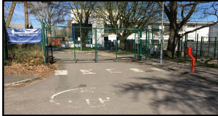
Picture 3-18 - Access Control Gates into Piper Hill Post-16 Educational Building
