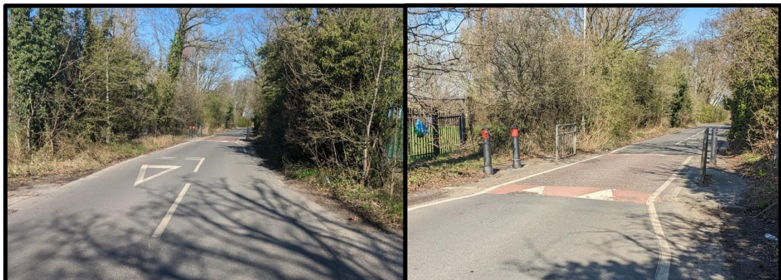
Picture 3-12 and Picture 3-13 – Pedestrian Crossing Buildout and Speed Calming measure
