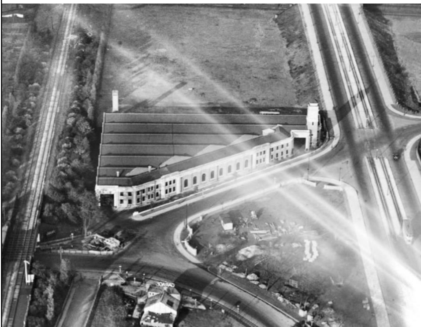
Figure 2: Oblique aerial view of Parrswood Bus Depot, pictured c.1929. The aerial image provides further detail on the original extent and layout of the Bus Depot, illustrating the clock tower formed a very minor component of the site.
