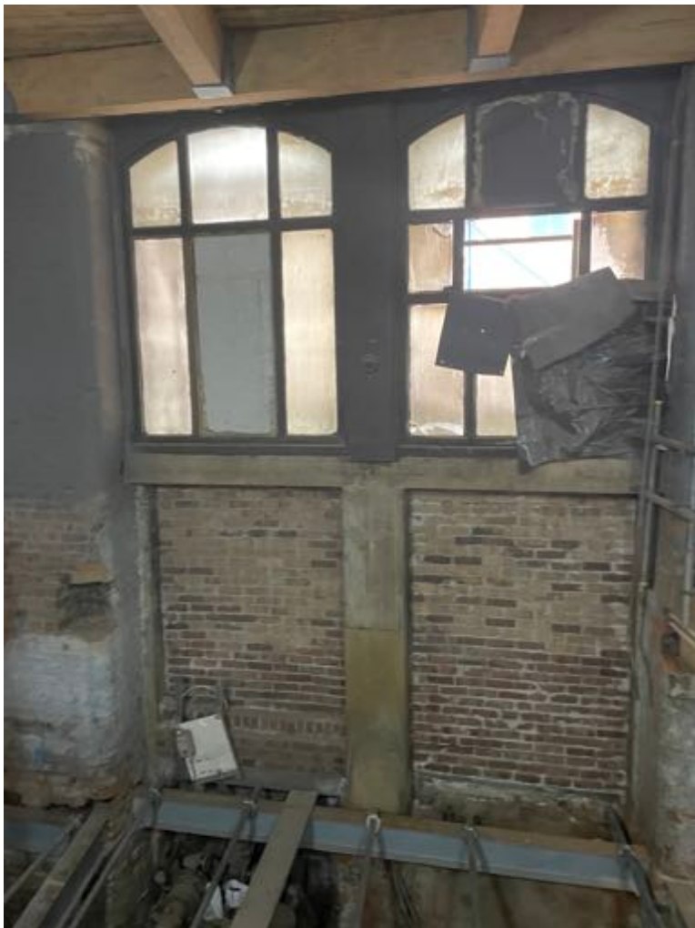
Stone frame bricked up
