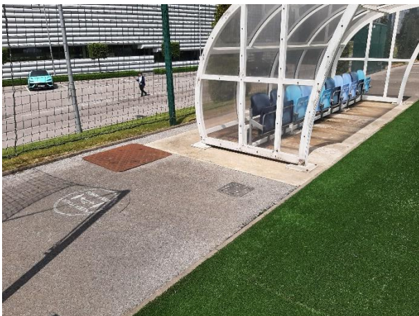
Photograph 3: Dugout, inspection covers, and mixed asphalt, artificial turf and concrete surface.
