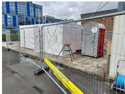
Photograph 3: Existing building on site.
