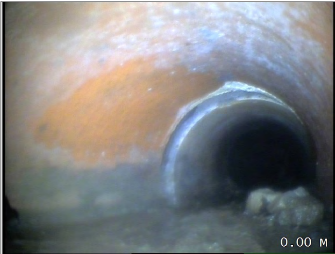
Start node type, manhole, reference MH 12
