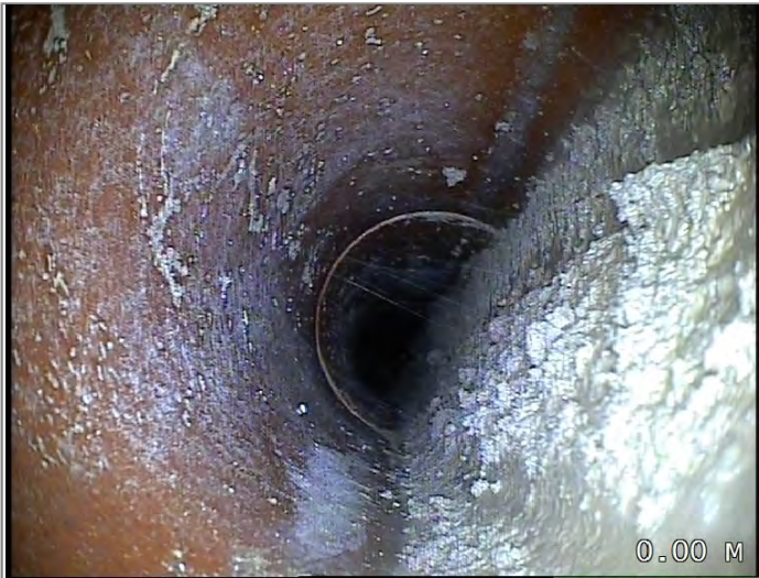
Start node type, manhole, reference MH 12
