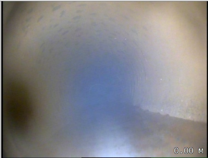
Start node type, manhole, reference MH 10
