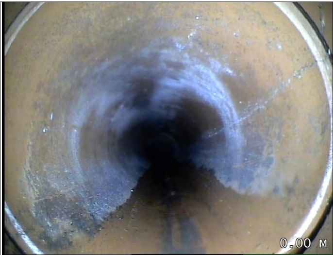
Start node type, manhole, reference MH 11
