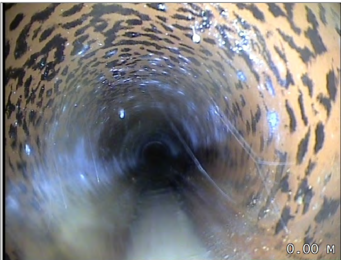
Start node type, manhole, reference MH 10
