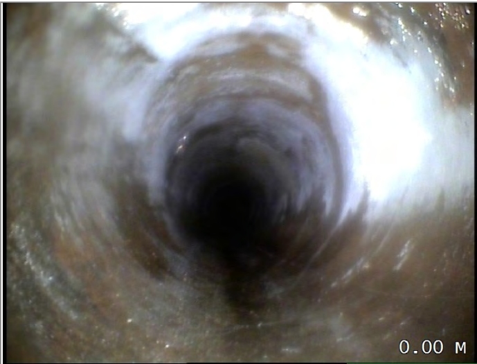
Start node type, manhole, reference MH 13
