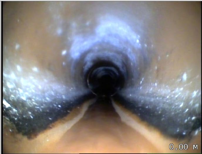
Start node type, manhole, reference MH 11
