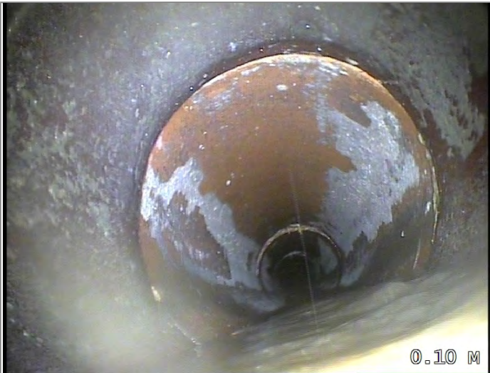
Start node type, manhole, reference MH 08
