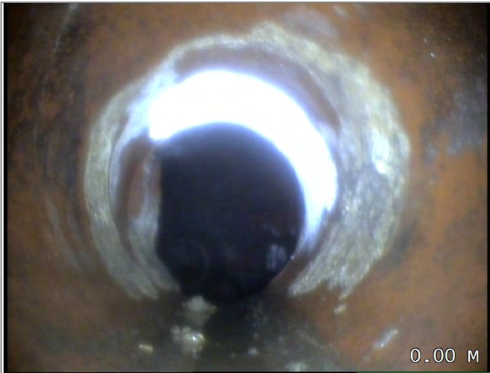
Start node type, manhole, reference MH 13
