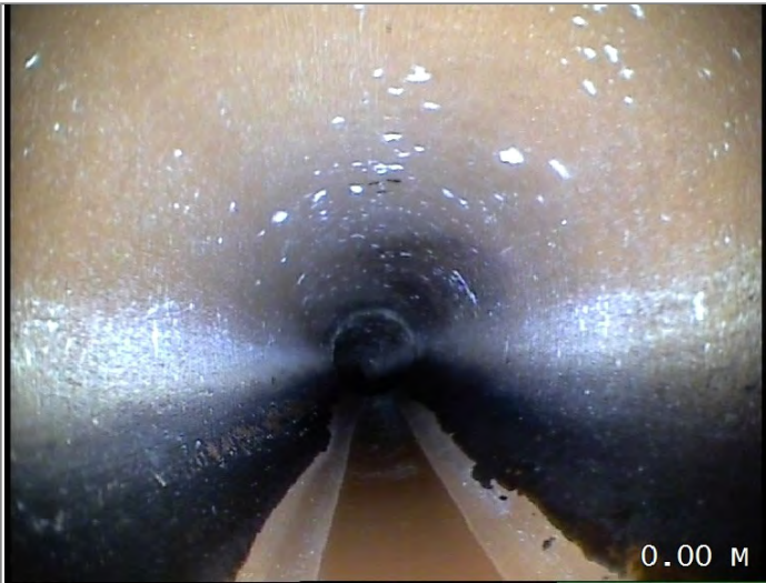
Start node type, manhole, reference MH 11
