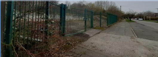
Steel railings and gates define the site's Longhurst Road boundary
