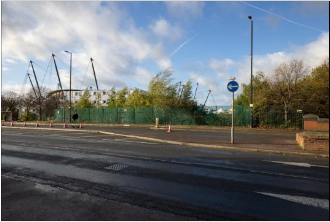
Figure 3.1 – Existing view Southwest on Alan Turing Way (Adjacent to Lock Keepers Cottage)
