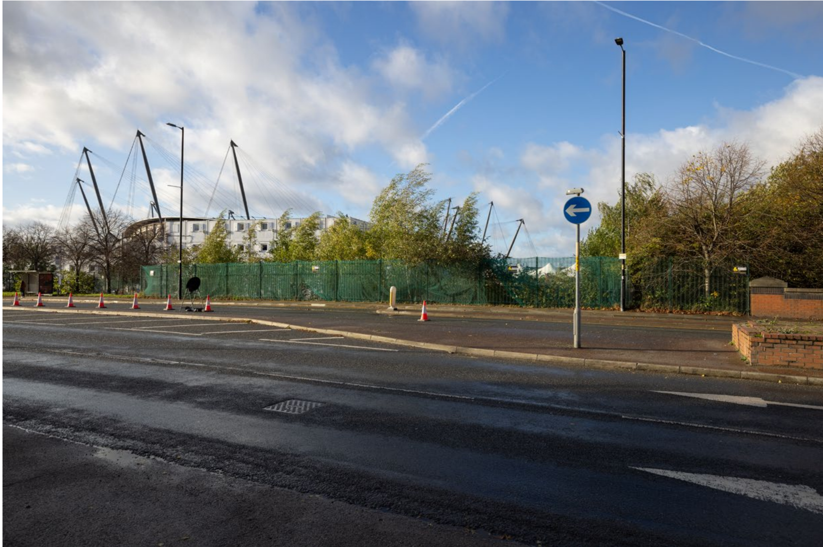
View 2: Baseline | View south west from footpath entrance to canal and Alan Turing Way - adjacent to Listed Lock Keepers Cottage.
