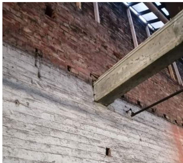
1. Existing beam below existing joists and exposed brick
