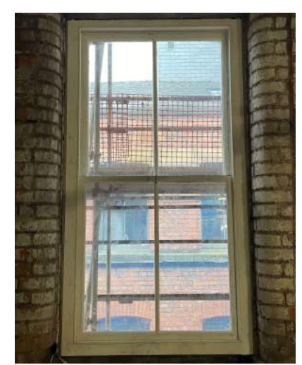
Photo of existing sash window along Mangle Street to be replicated.
