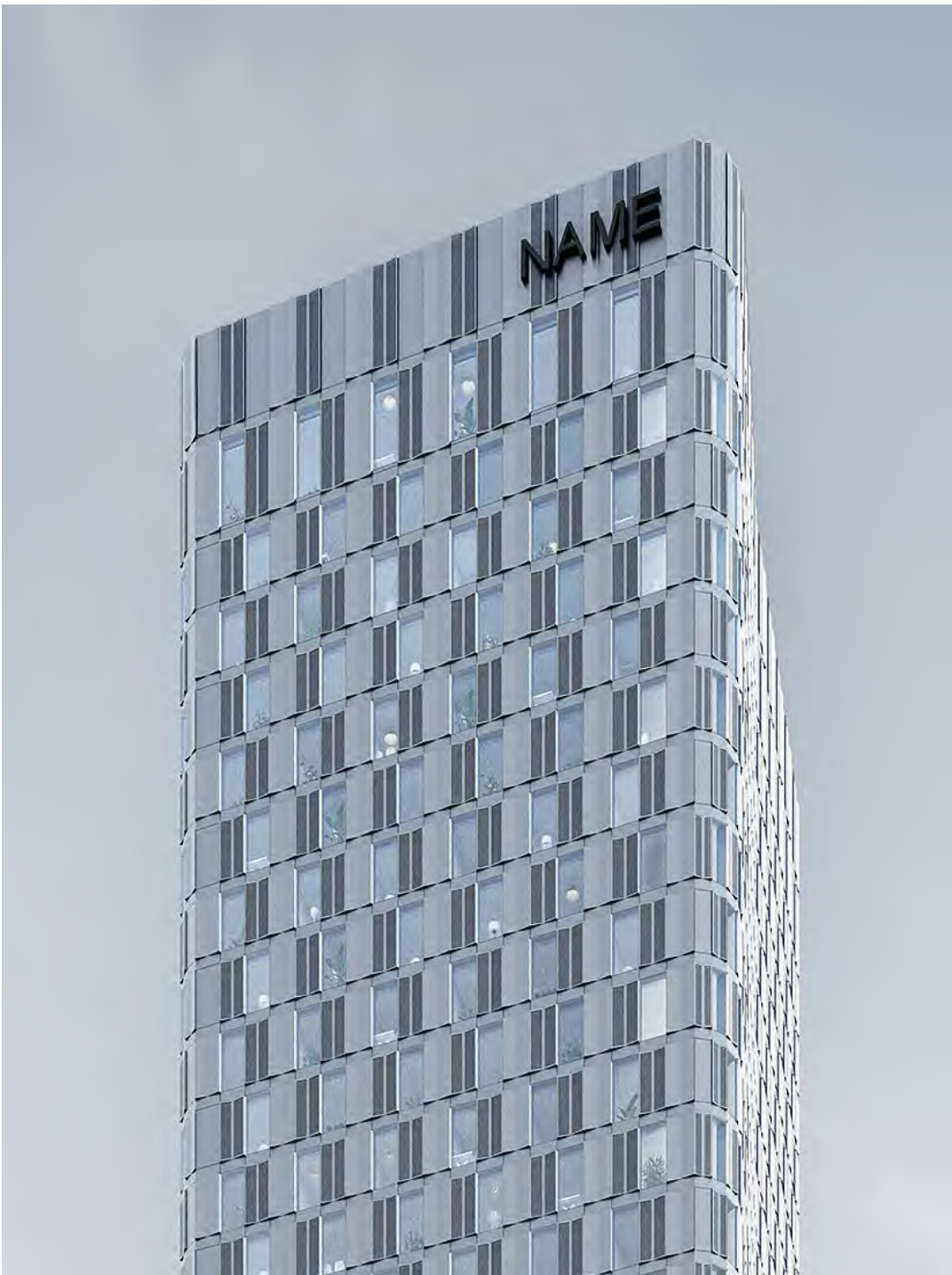
Building A1 parapet signage
