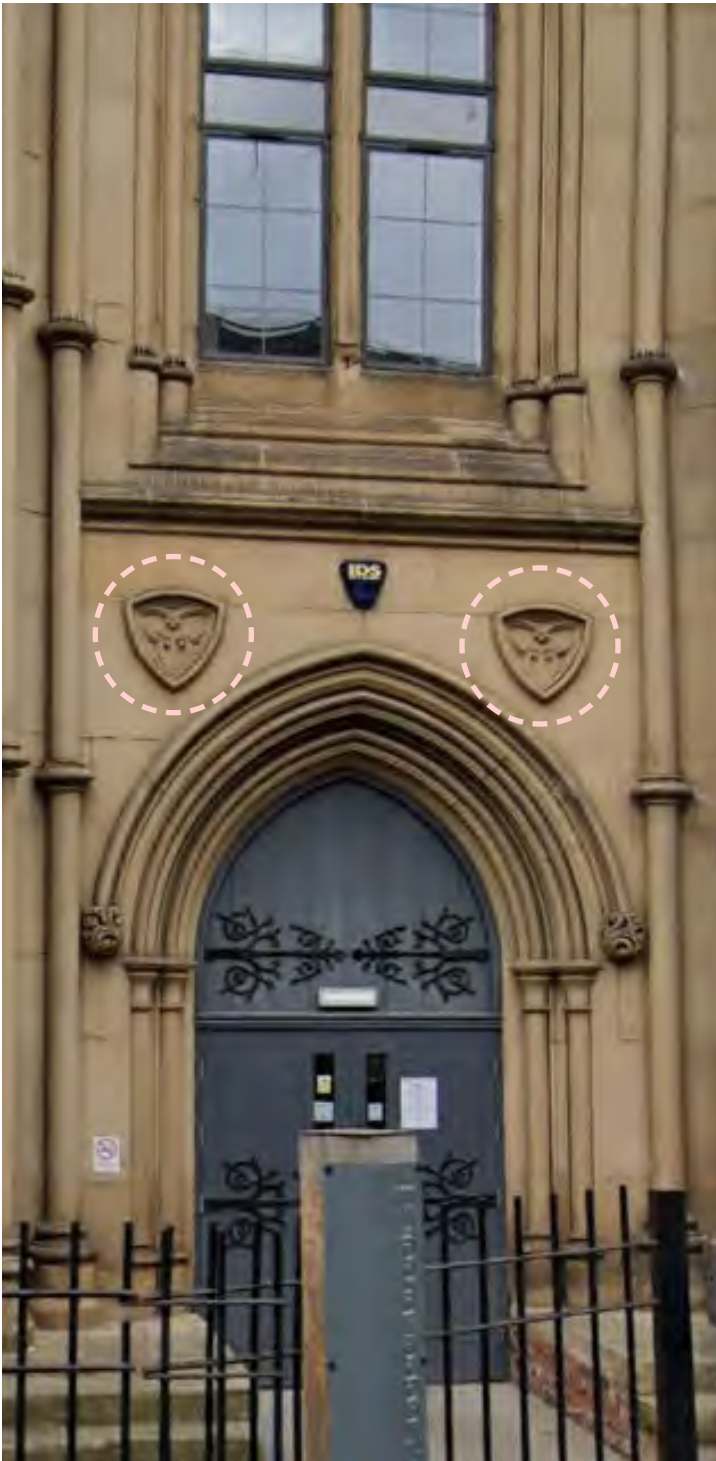
Mouldings on adjacent listed chapel
