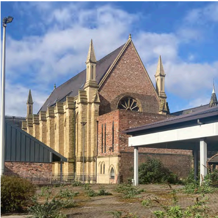
Rear (East Elevation) of Chapel
