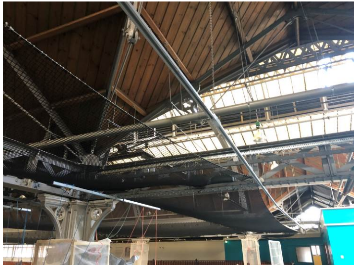
Figure 32: Central section of the eastern side of the roof structure, showing the 1980s timber boarding replacements.
