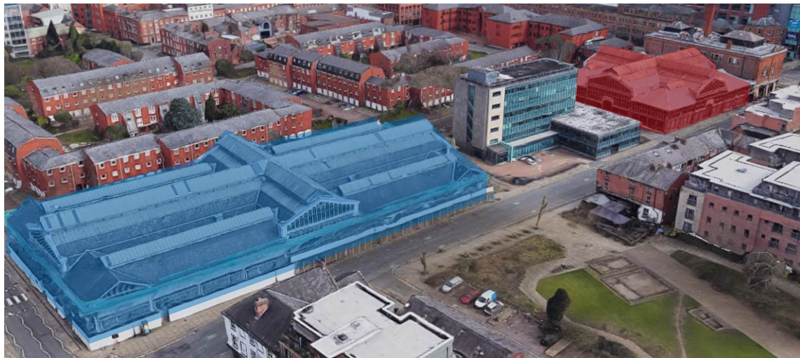
Figure 1: An aerial view looking north-east across the Lower Campfield Market (The Site - shaded blue) and Upper Campfield Market (shaded red – not part of this assessment) (Source: Google).
