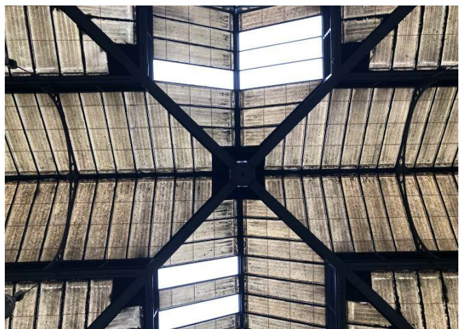
Figure 33: An example of the modern 1980s fibreglass panels (discoloured) and more recent clear coverings.
