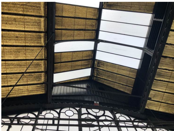
Figure 33: An example of the modern 1980s fibreglass panels (discoloured) and more recent clear coverings.
