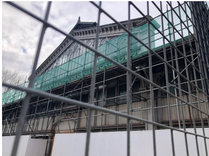
Figure 24: The east elevation.
