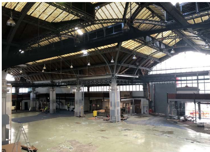
Figure 27: Looking south-east across the building towards the southern elevation.
