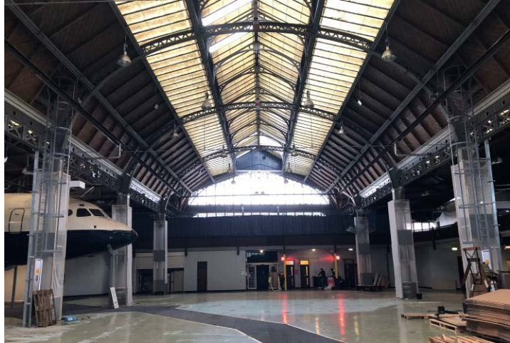
Figure 29: Looking west across the building towards the north elevation.
