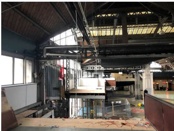
Figure 36: Looking west along the southern mezzanine
