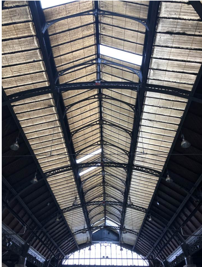
Figure 35: Looking west along the length of the roof structure.
