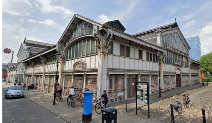
Figure 23: The south elevation (left) and east elevation (right) (2018)
