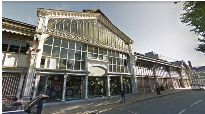
Figure 17: The central, raised portion of the southern elevation, showing original cast iron Venetian windows to gable and modern glazed openings to lower portions in the place of removed original cast iron railings. (2018)
