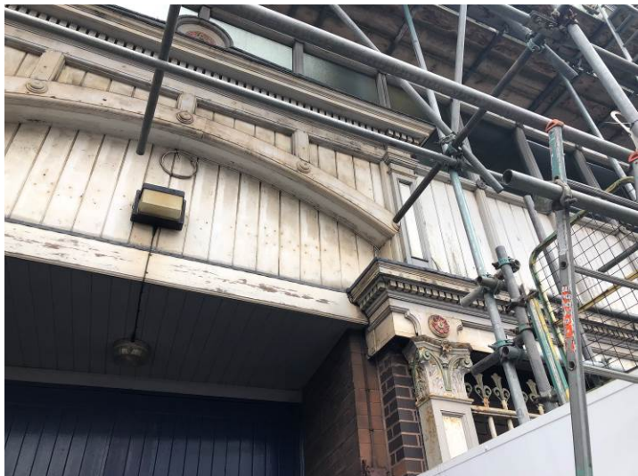
Figure 22: The lower parts of the west elevation.
