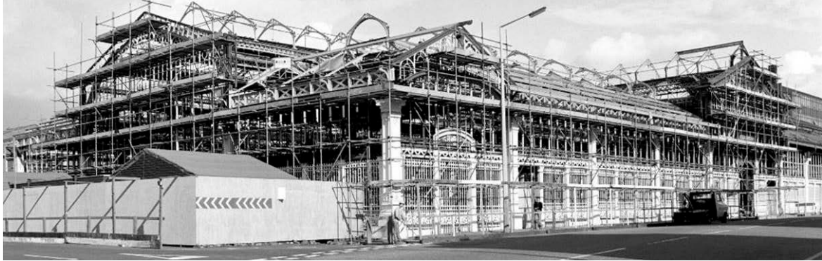
Figure 14: The Lower Campfield Market building during its substantial renovations in 1981 in preparation for becoming the Manchester Air & Space Museum. Note the complete removal of roof and elevation coverings. (Source: Manchester Archives).
