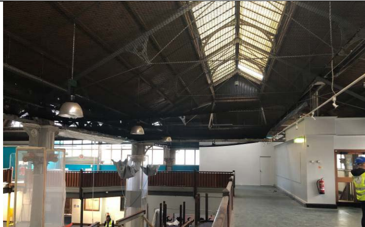
Figure 37: Looking east along the southern mezzanine.
