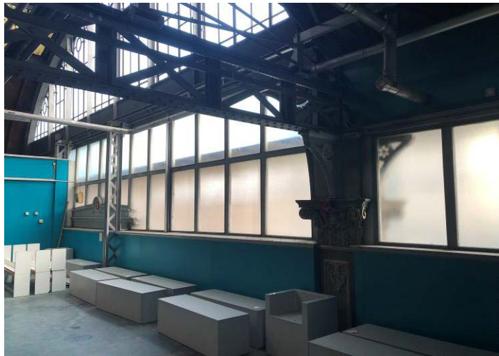
Figure 38: The eastern side of the southern mezzanine.
