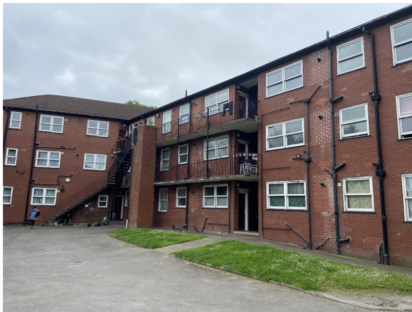
Views of the rear elevations from the car park
