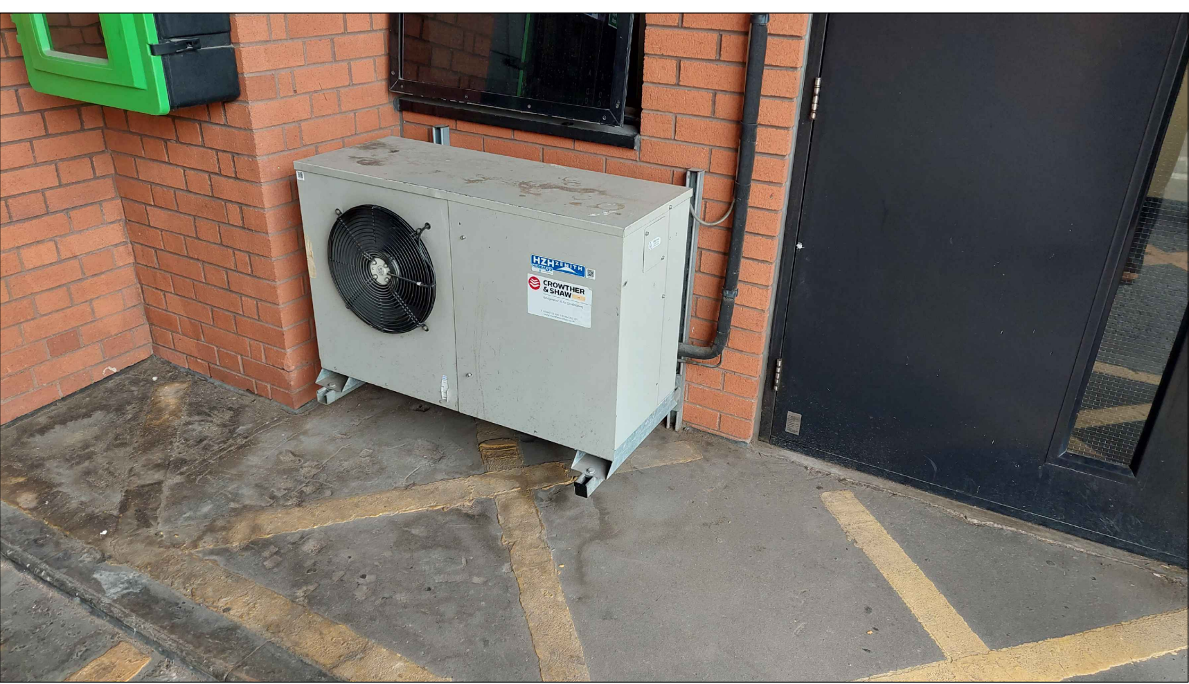
PHOTO 3 - EXISTING 1NO. COLD CONDENSER TO BE REPLACED FOR NEW. NEW SUPPORT FRAME SHALL BE INSTALLED IN THE SAME POSITIONS AS EXISTING.
