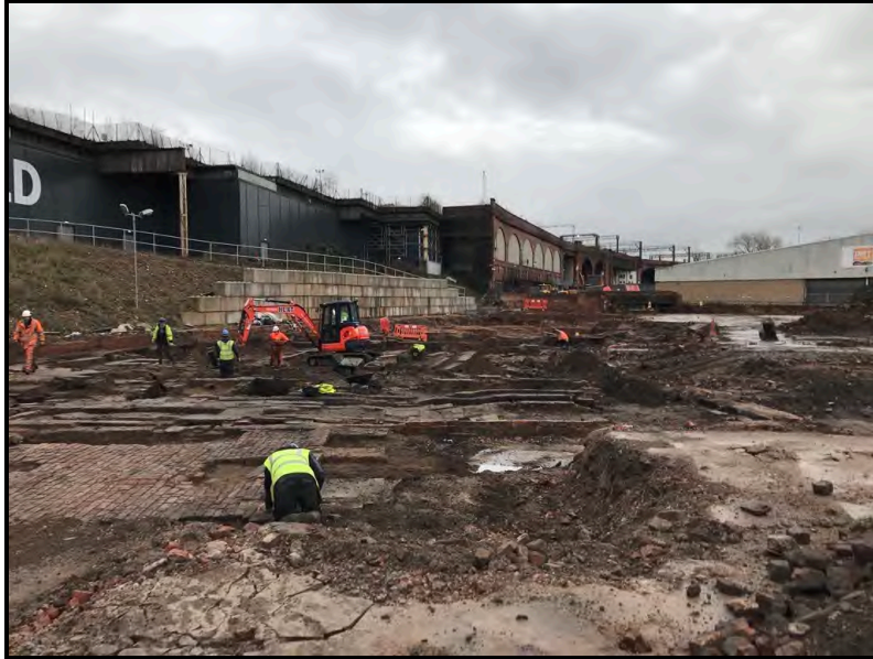
Plate 2.2: Chapelfield Dye Works Excavations
