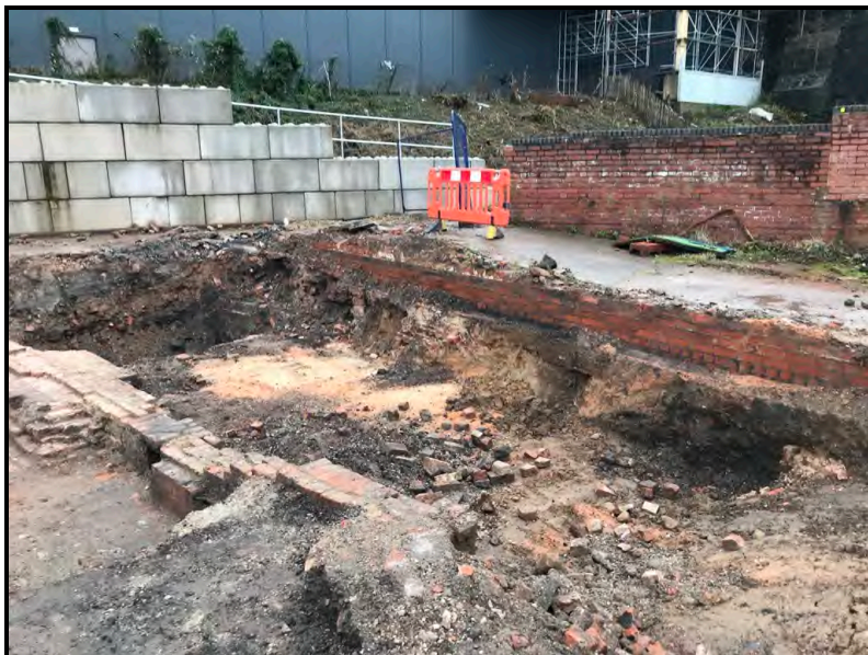
Plate 2.1: Chapelfield Dye Works Excavation
