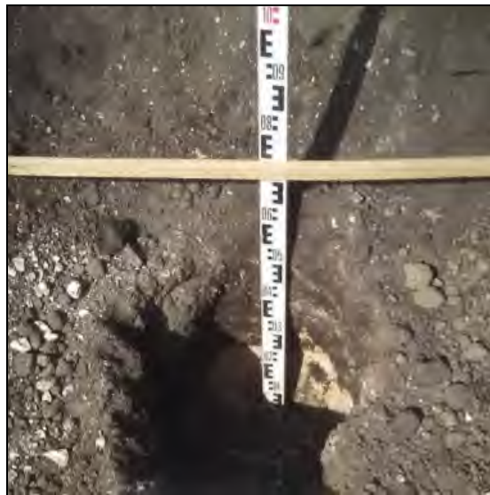
Fig 3.0 Example of soil capping depth validation photograph
