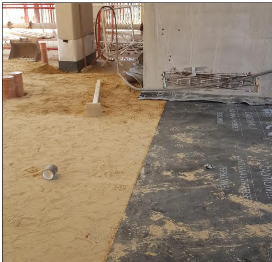
Figure 1: Photo showing the sand blinding layer prior to the membrane installation
