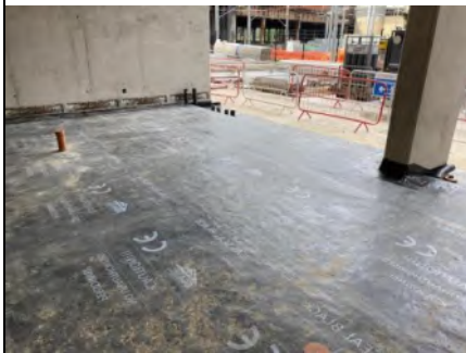
General Overview of gas seal black application, all laps correct and sealed well.
