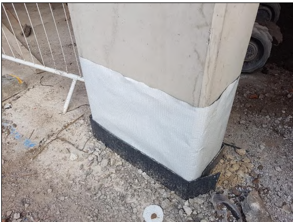
Figure 3: Photo showing area prior to installation
