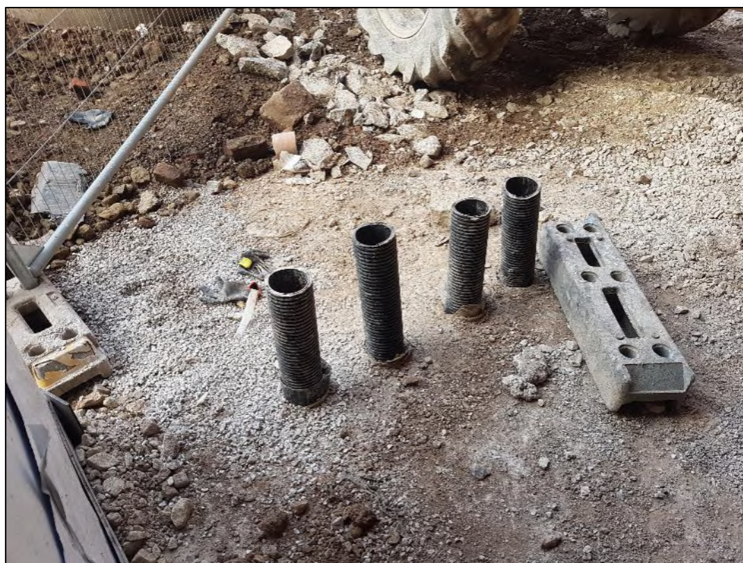
Figure 4: Service ducts prior to installation
