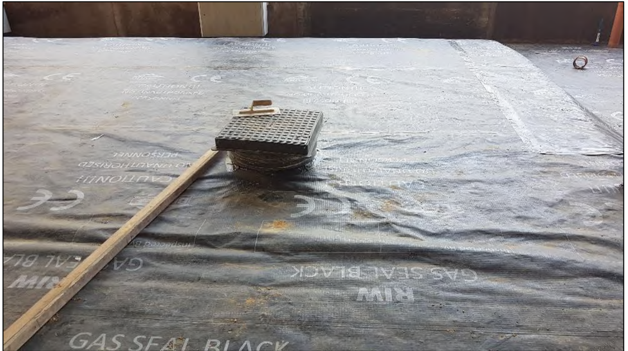
Figure 9: Membrane installation with manhole penetrations
