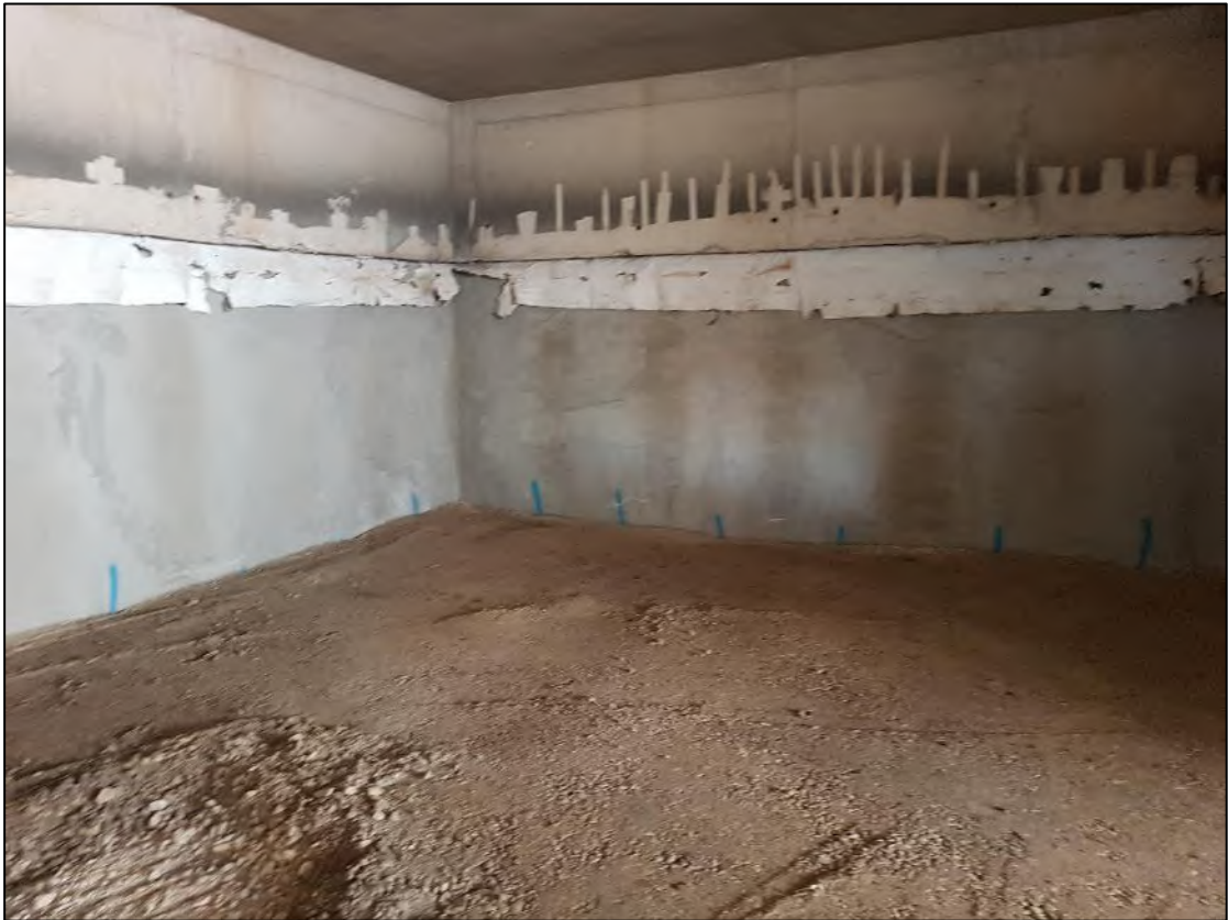
Figure 1: Photo showing SE area prior to installation
