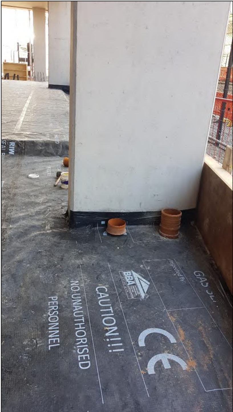
Figure 6: Membrane installation along building edge, service penetrations and columns
