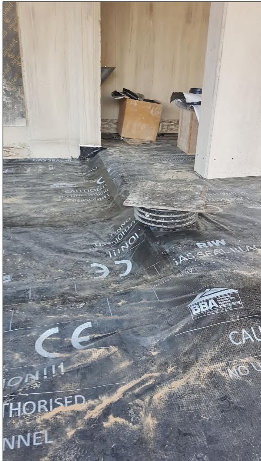
Figure 7: Membrane installation with manhole penetrations prior to completion
