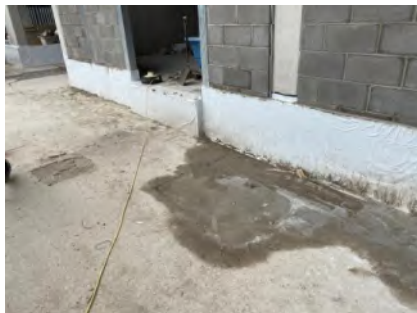
Sheetseal GR applied with block work installed on top of upstand.
