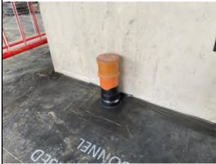
Pipe penetration detail sealed with top hat.
