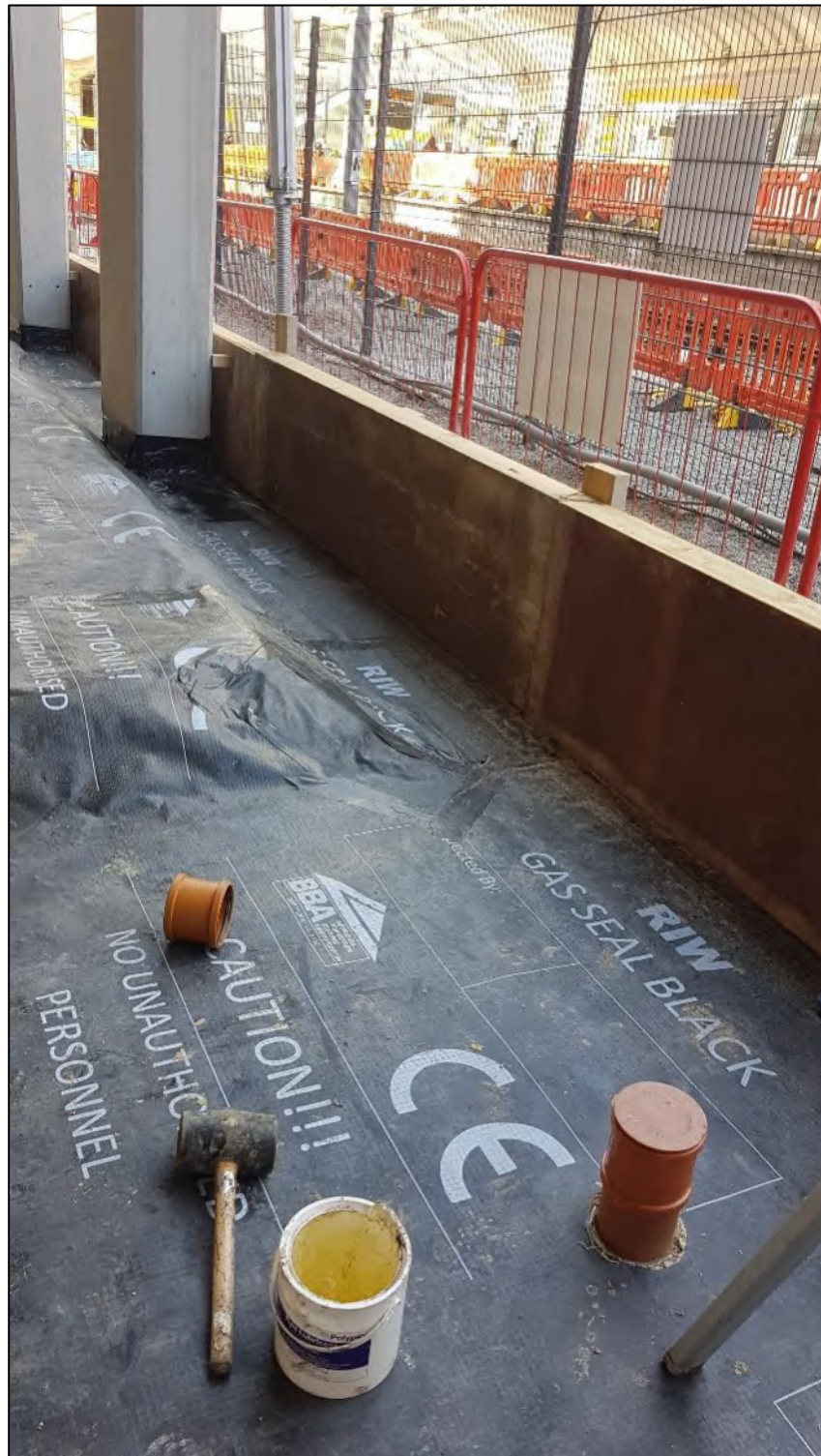
Figure 5: Membrane installation along building edge and columns
