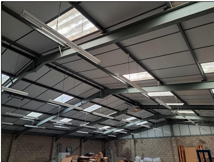
Photograph 9 showing the internal roof
