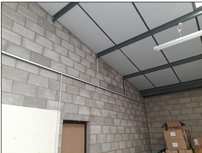
Photograph 11 showing the metal beams
