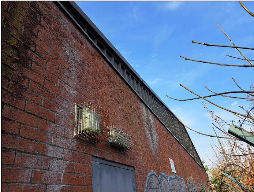
Photograph 8 showing the gable end
