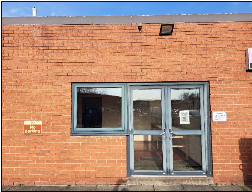
Photograph 6 showing the doors and windows
