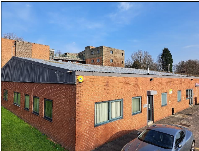
Photograph 7 showing the roof
