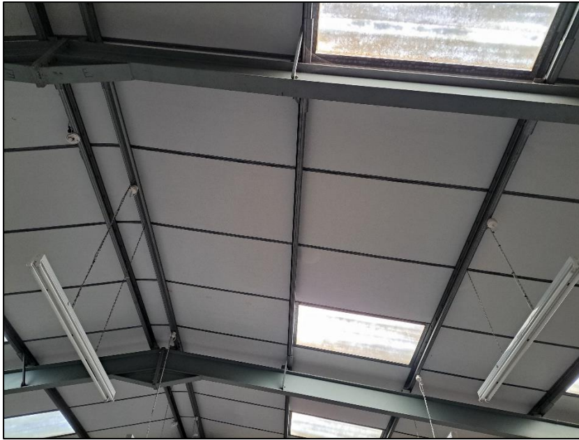
Photograph 10 showing the underside of the roof
