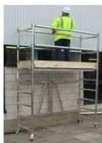
Low-level Access tower <2.5metres
