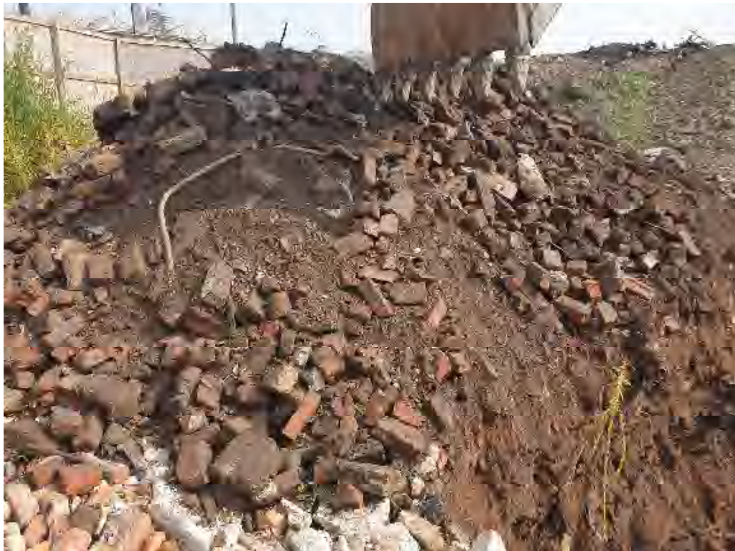
Photo No. 2: TPI01 Arisings
