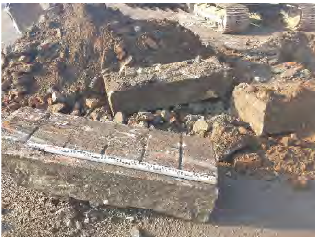
Photo No. 10: TPI04 Arisings
