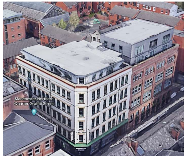
Photo – 2 adjacent buildings along Tib Street
