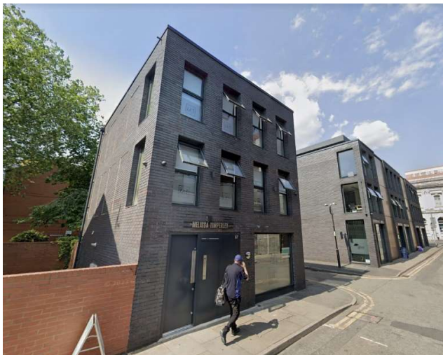
Photo – Recent development along Tib St. with the same external appearance to the proposed application site.
