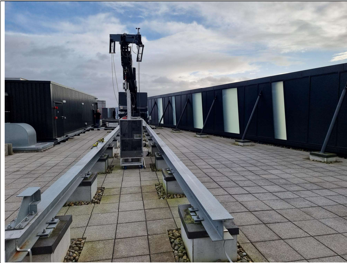
Figure 1 – Roof finishes topped by 80mm thick concrete paving flags
