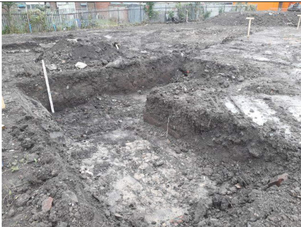
Photograph of Trench 1 excavation in the location of WS102. Edge of the former pond can be seen in the top left of the photograph.
