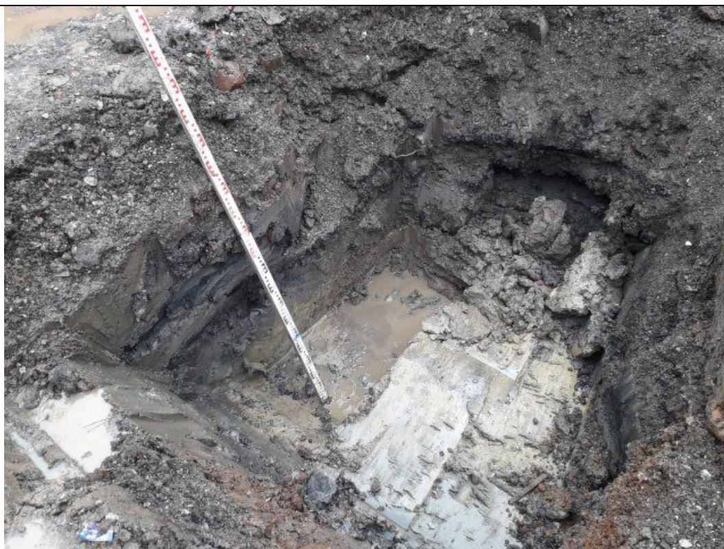
Delineation excavation in the location of TP201. Clean clay shown at the base.
