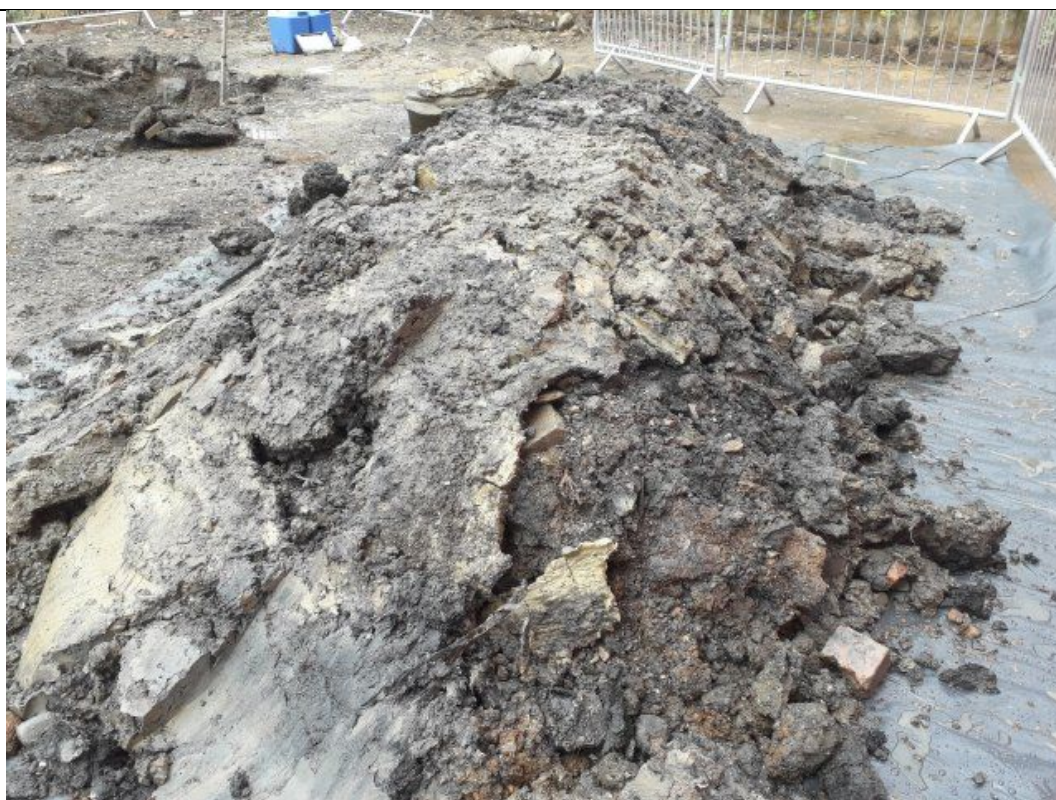
Material excavated from TP201 stockpiled on Visqueen. N. B. Visqueen lapped up and stockpile covered once excavations complete.
