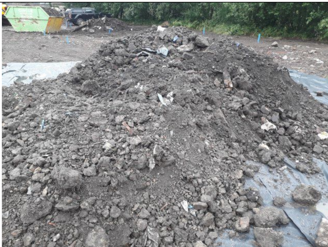
Stockpile of excavated contaminated material from around WS102. N. B. Visqueen lapped up and stockpile covered once excavations complete.
